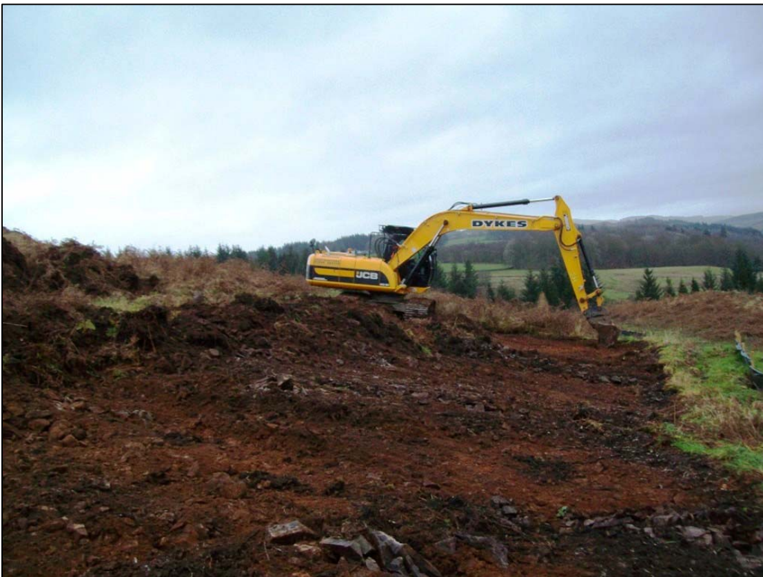
Figure 3b: Mechanical excavator stripping lower eastern area of site.
