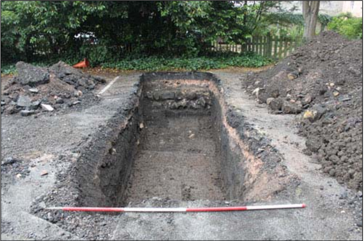
Figure 4a: Trench 1 from the East
