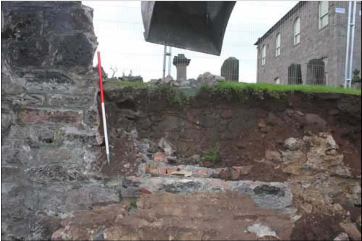
Figure 5a: Wall 003 and modern brick repairs revealed behind Retaining Wall 000
