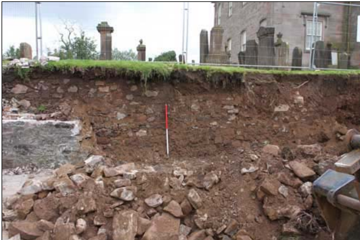
Figure 6b: Retaining Wall 002 Revealed following removal of Deposit 003
