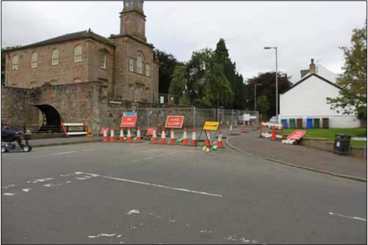
Figure 4a: General View, Showing Modern Church with Retaining Wall to north
