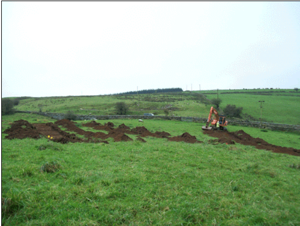
Figure 3a: General shot of site from the northeast with Trenches 3, 4 and 5
