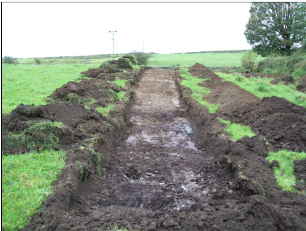
Figure 4b: Trench 2 from the east-north-east
