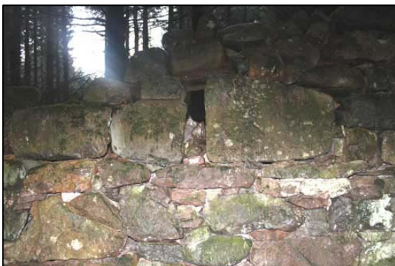
e: Detail of Window, Structure 1004
