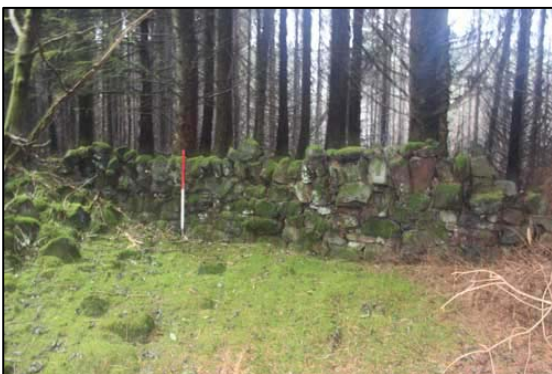
g: Rear (N) Wall of Room C, 1002
