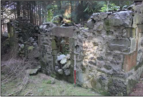
a: Exterior View From S, (1001)
