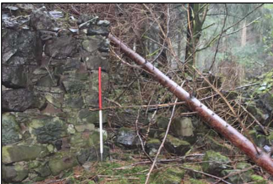
e: Doorway, SE Wall, Room A (2001)
