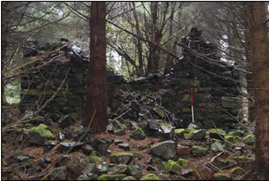
c: Structure (2001), SW Gable Wall
