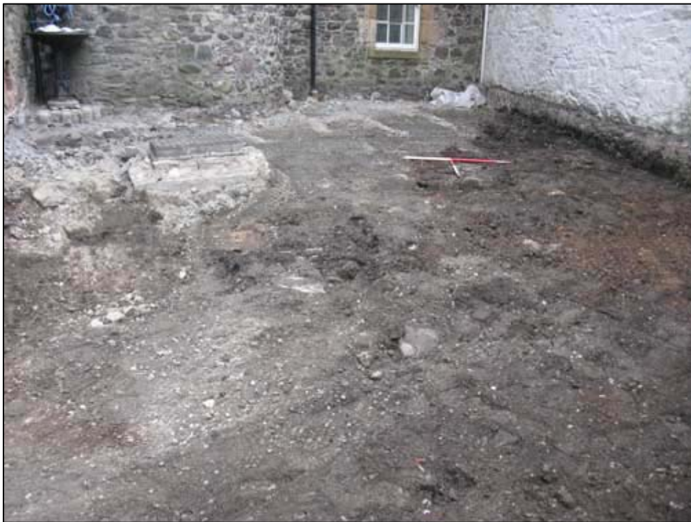
Fig. 5b: South Extension – Fully Excavated
