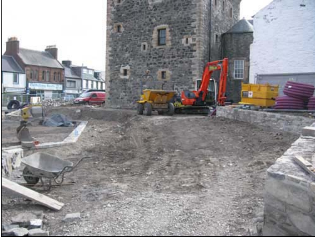
Figure 5a: General View of Site, Showing Works in Vicinity of Tower-House
