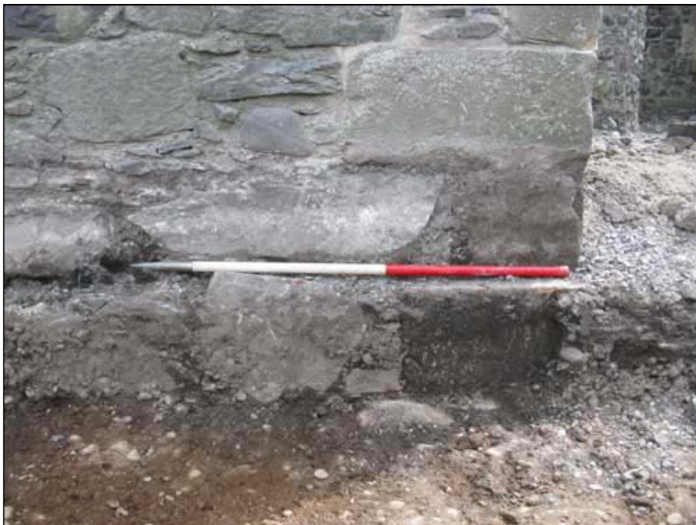
Figure 5b: Basal Course of Masonry (009) revealed at foot of Tower-House
