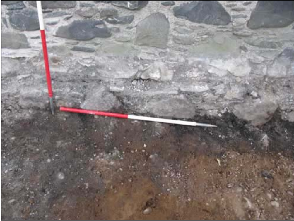
Fig. 8a: Foundation Trench [014]/(015), with later cuts evident: [018]/(019) to left, [022]/(023) to right
