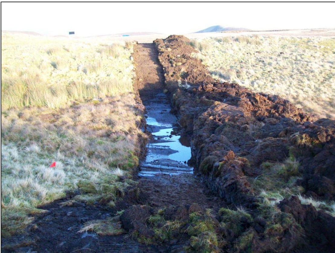
Figure 5b: Trench 7 from the west.
