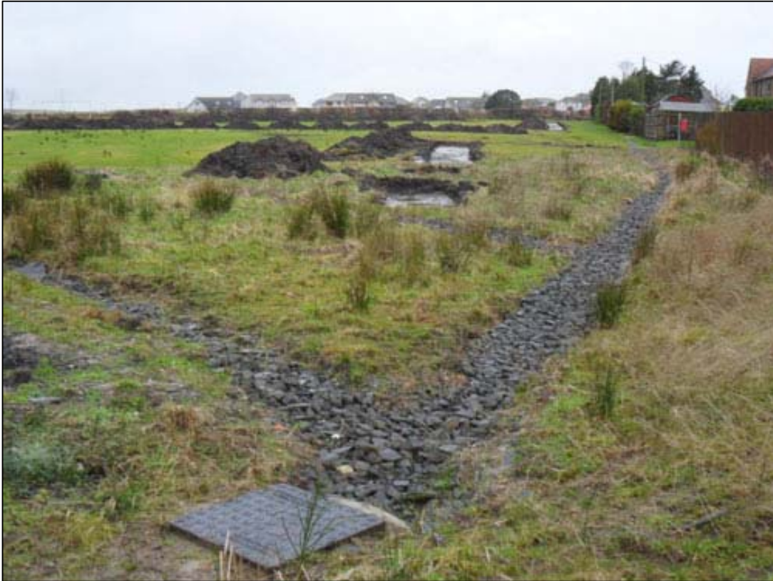
Figure 3d: North-east area of site (showing modern drains/manhole)
