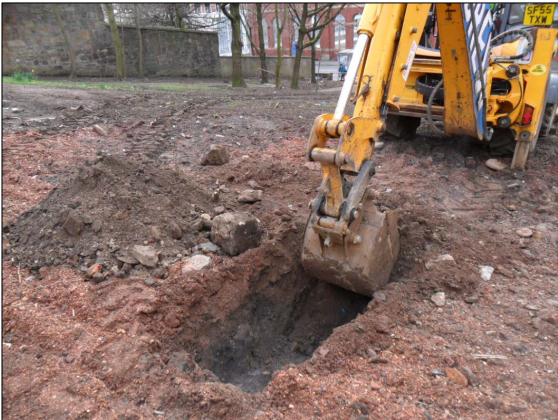
Figure 1b: Excavation of test pits prior to development
