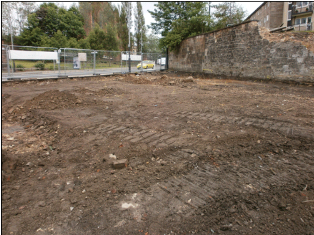
Figure 4b: North end of site, original wall and remodelled upstanding wall [022]
