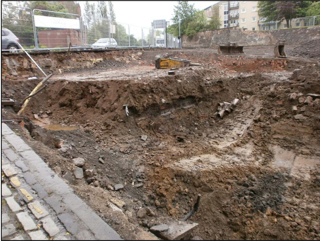
Figure 4a: Excavations at north end of site
