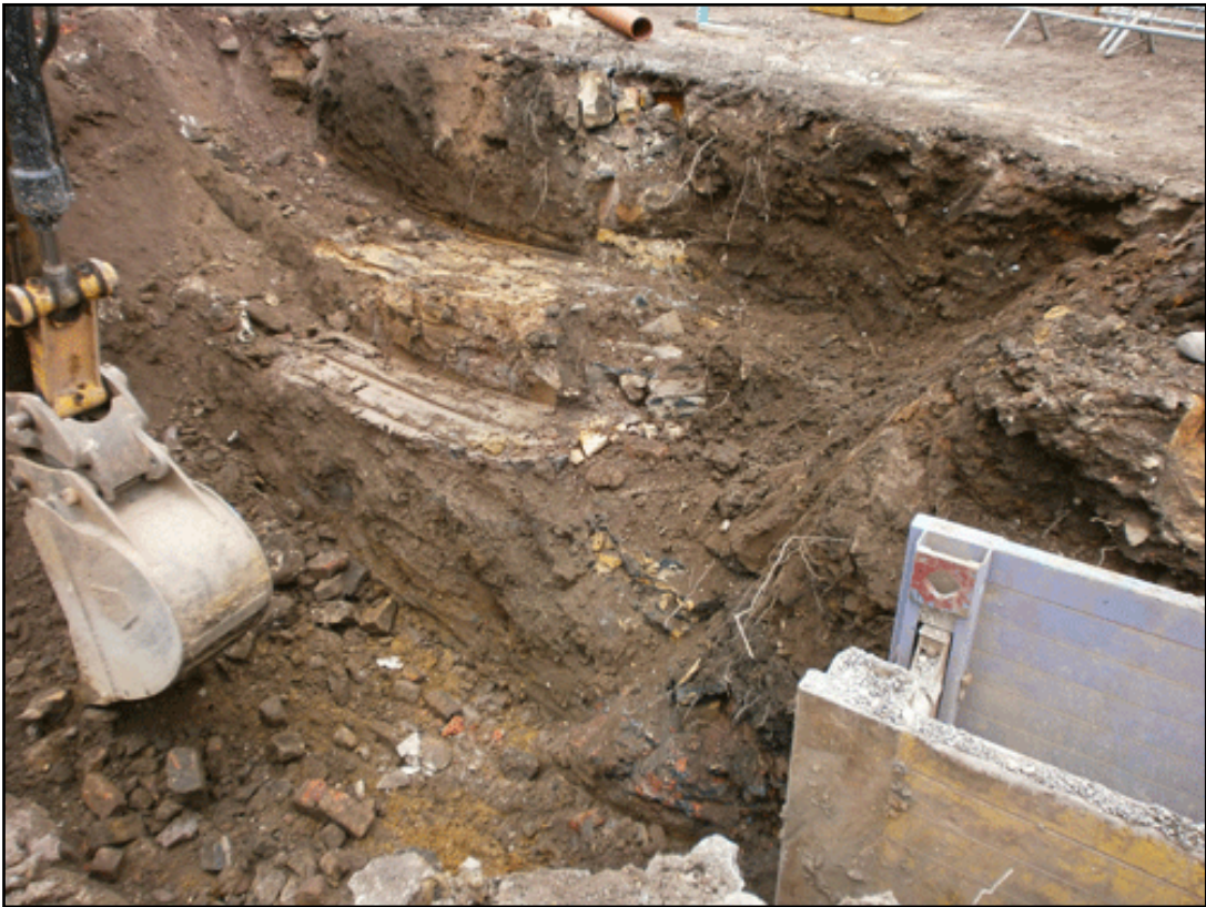
Figure 5b: Foundation of wall [022] (pipe trench)
