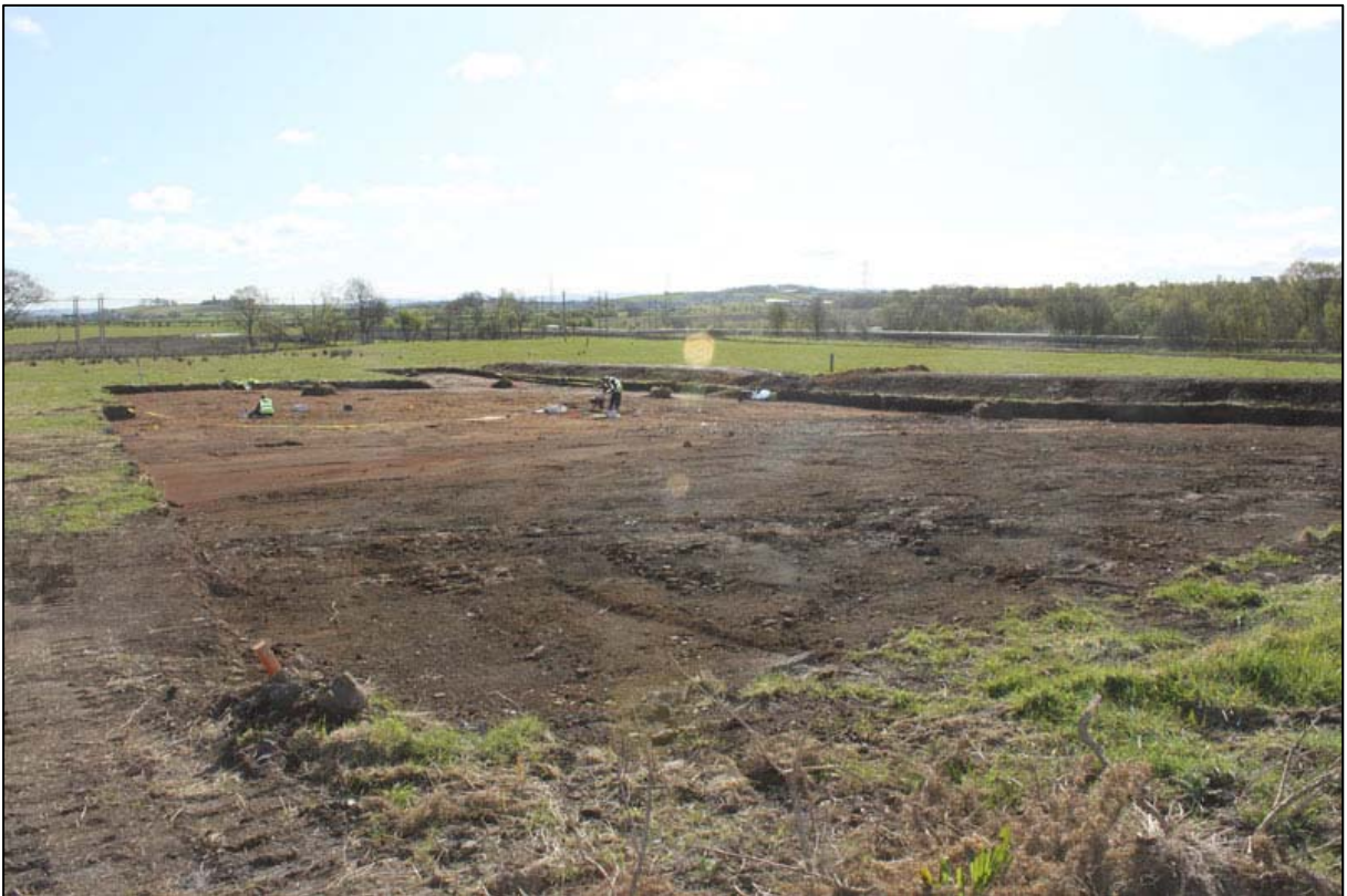
Figure 4b: General shot of Turbine 3 area from the northwest
