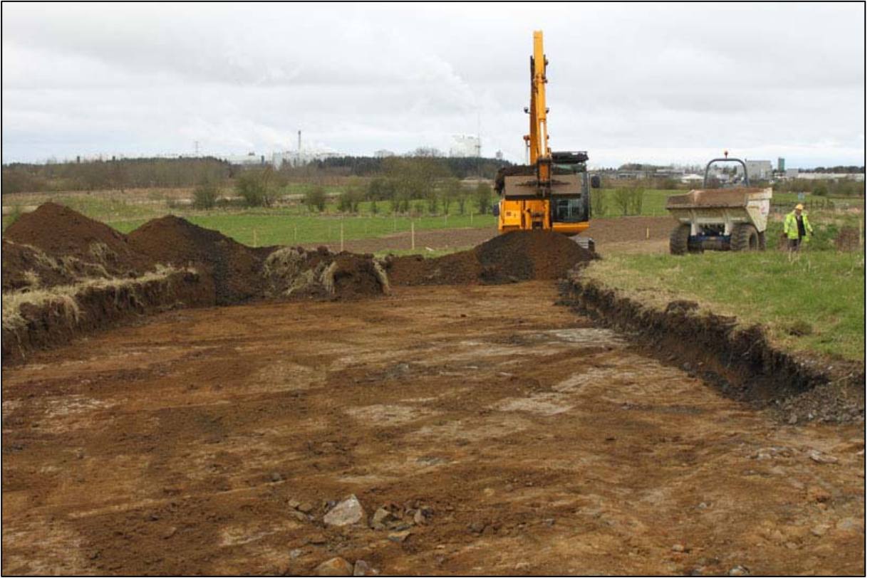
Figure 2a: Groundbreaking works for Haul Road 3 from the east
