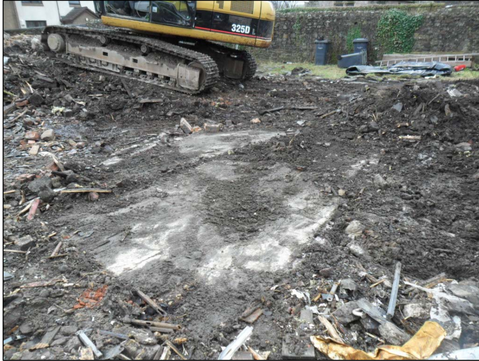
Figure 3a: Showing the concrete base (003) before removal
