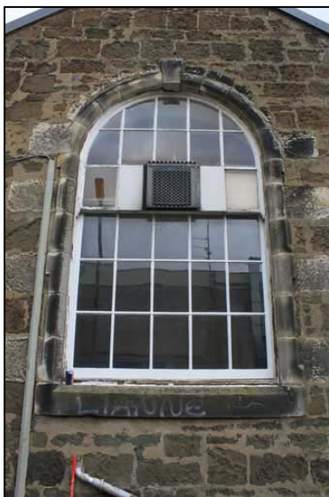
Fig. 8e: Arched Window, W-Facing Elevation, N End
