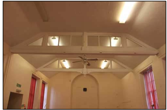
Fig. 11b: Room g, Glazed Panels in Roof Truss
