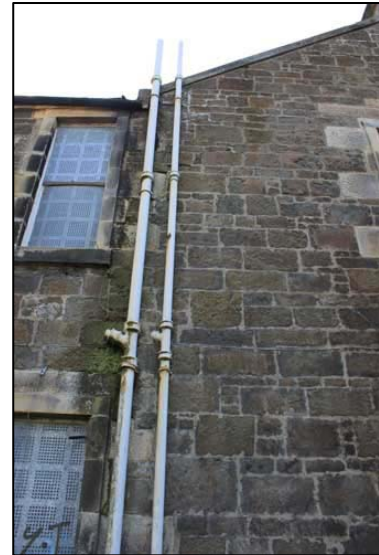
Fig. 4b: Police Station, S Elevation possible Running Joint
