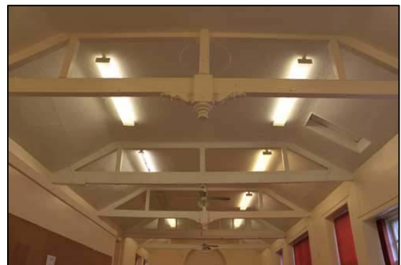
Fig 10f: Room g, Detail of Roof Trusses
