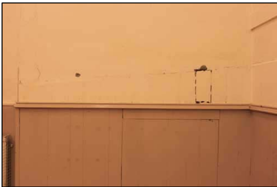
Fig. 11e: Room g, Panelling at S end
