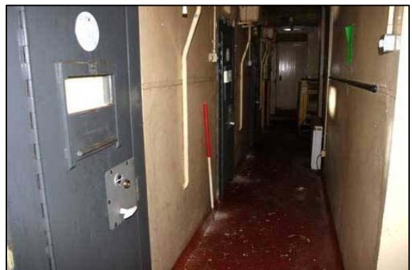
Fig. 6f: General View of Cell Bay
