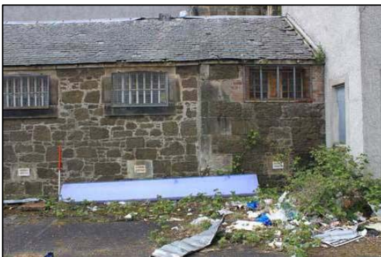
Fig. 4e: Police Station, N Elevation, visible Phasing in Cell Block
