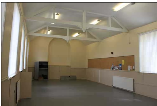
Fig. 10e: General View, Room d
