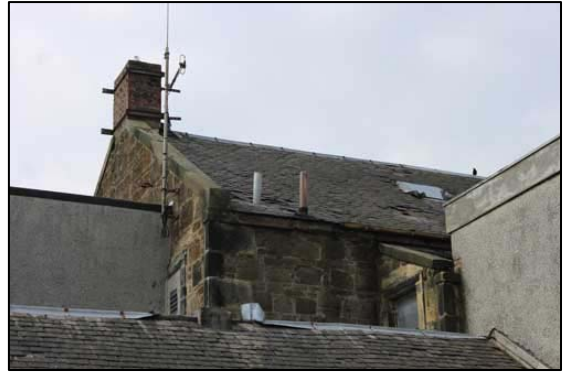
Fig. 6b: Exposed Upper Storey, with Projecting Stair
