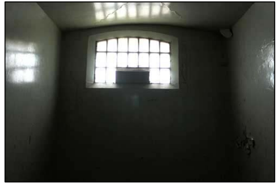
Fig. 7d: Window in Segmental Arched Setting (Cells i - iv)
