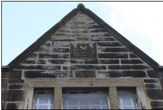
Fig. 3c: Police Station, S Elevation Armorial Panel over 1 st floor window
