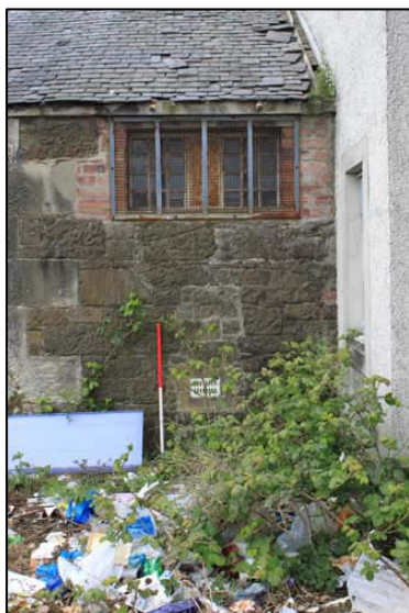
Fig. 7e: Alterations to Window, exterior of Cell v
