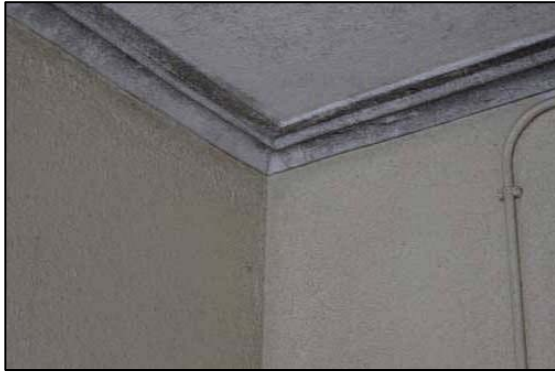
Fig. 6a: Example of Original Cornice, Room d
