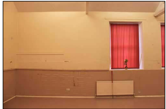
Fig. 11d: Room g, Panelling at S end
