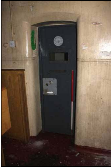
Fig. 7a: Recessed Cell Door (Cell i), E end, Cell bay
