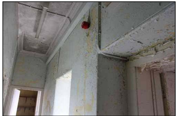
Fig. 6d: Cornice, N end Room i
