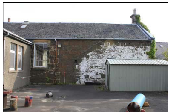
Fig. 11h: Site of Outbuilding, S Elevation
