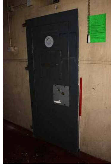
Fig. 7b: Cell Door Flush With Walls (Cells ii-v)
