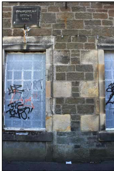
Fig. 3e: Police Station, W Elevation with blocked doorway
