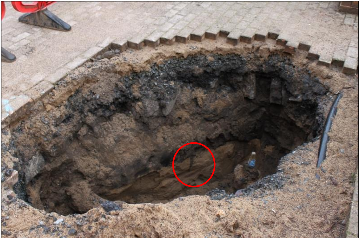
Figure 3: Western pit of Scottish Water works outside 57 to 63 High Street with truncated in situ soil profile visible under cobbles and over sand subsoil.
