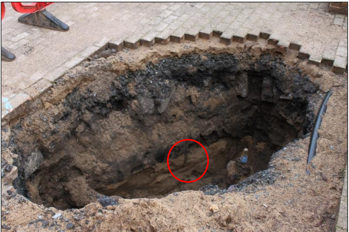
Figure 3b: Western pit of Scottish Water works outside 57 to 63 High Street with truncated in situ soil profile visible under cobbles and over sand subsoil.
