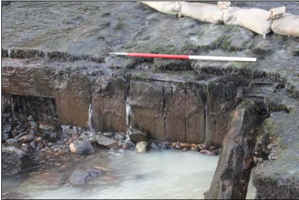
Figure 4a: Trench 1: In Situ Timber Shuttering on N side
