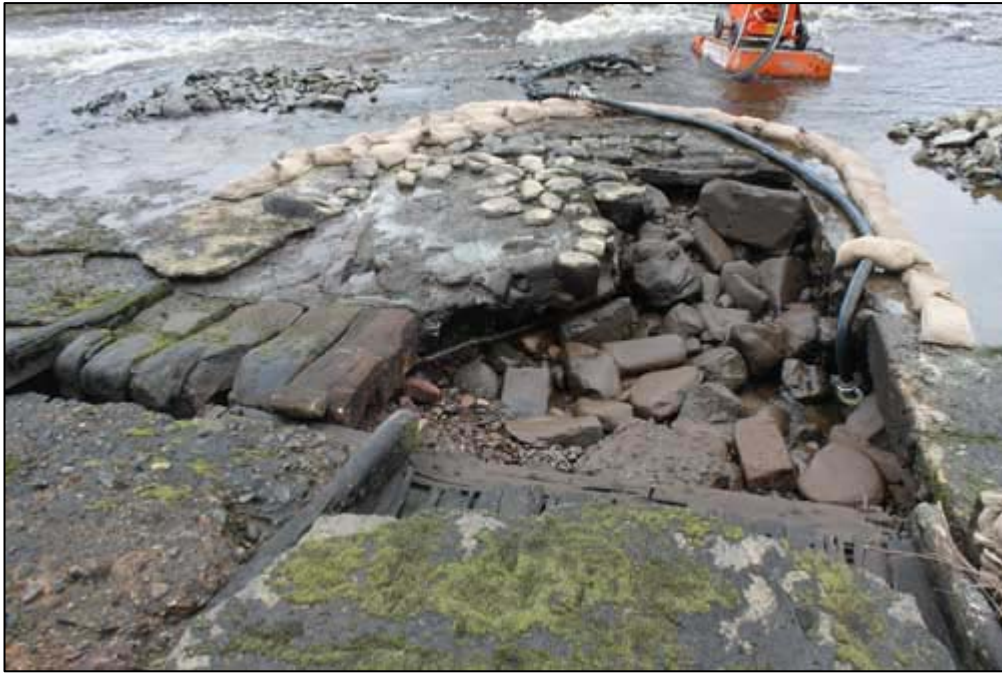
Figure 6a: View of Trench 3 from WNW, post-excavation
