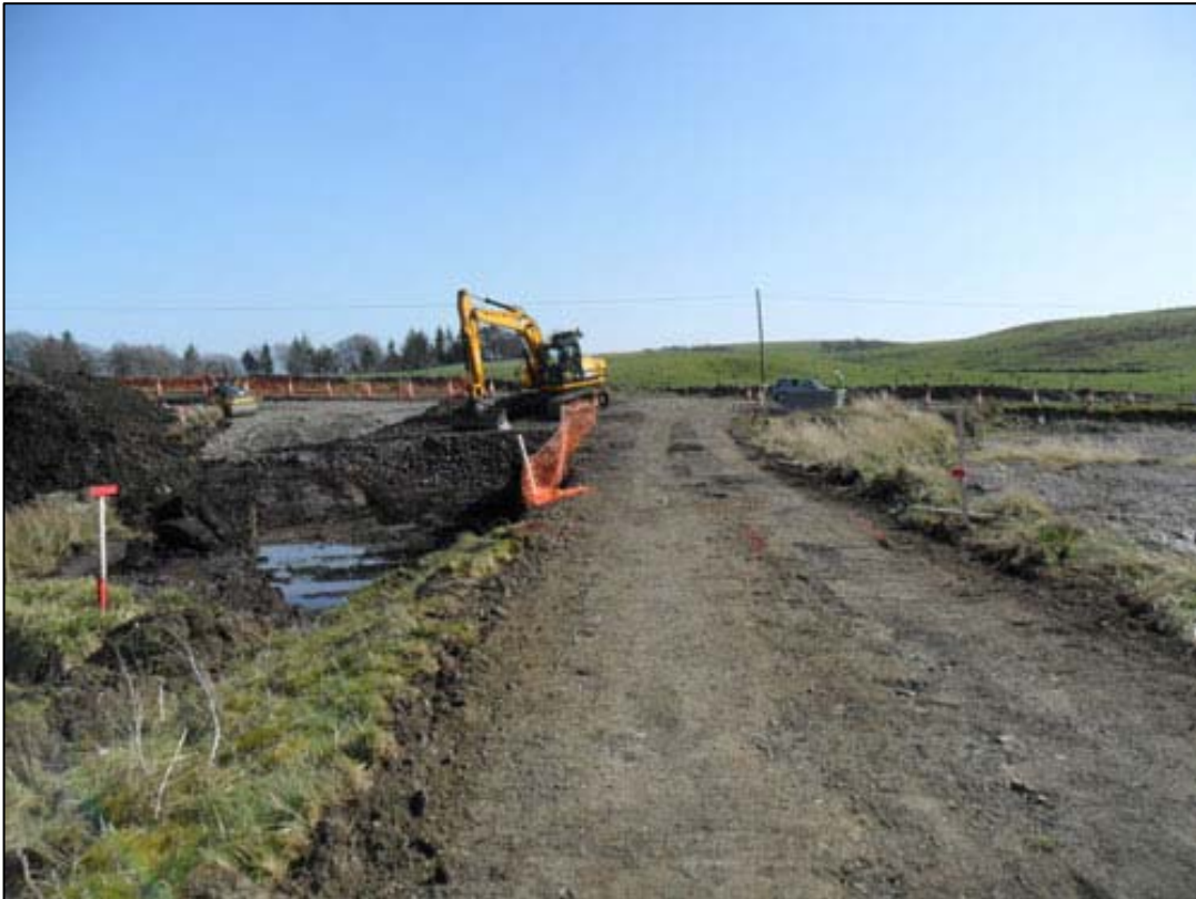
Figure 3a: Area 1 main entrance and bell-mouth
