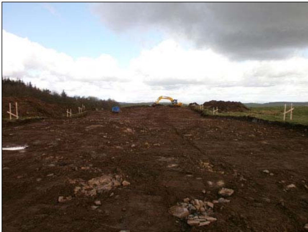
Figure 4b: Excavation of Area 4 main access road
