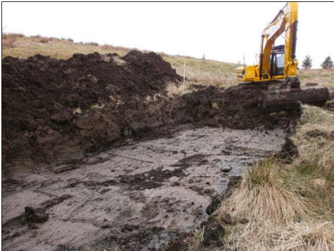
Figure 3b: Area 3 excavation of main access road
