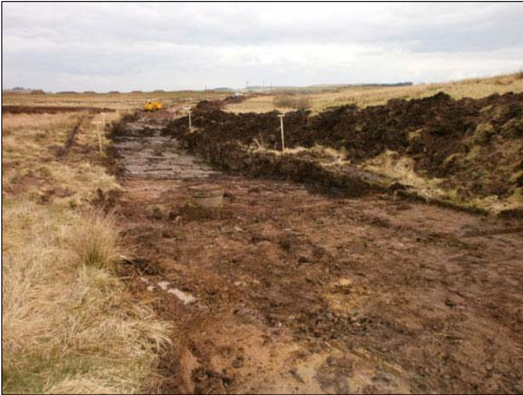
Figure 5a: Area of landfill cut by main access track within Area 3
