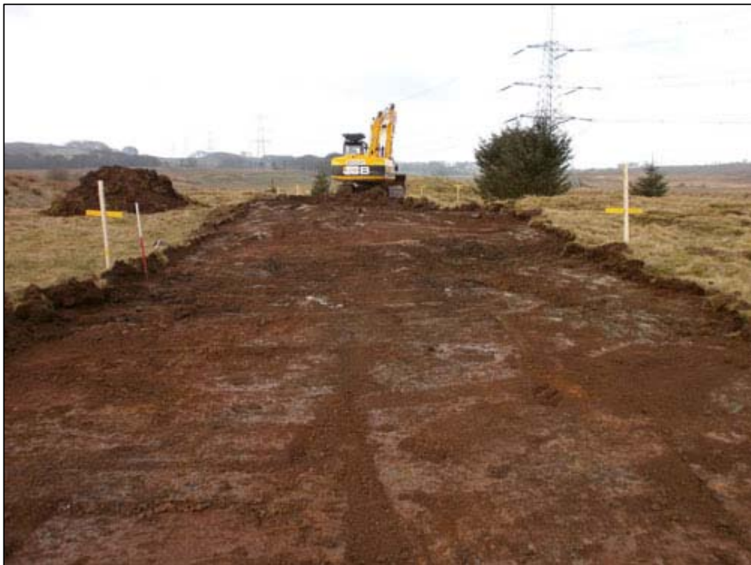
Figure 5b: Excavation of Area 5 main access track
