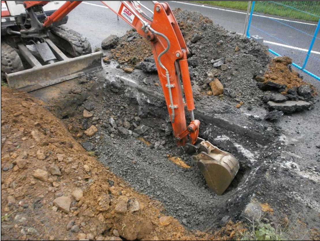
Figure 3a: Opening trench 047.
