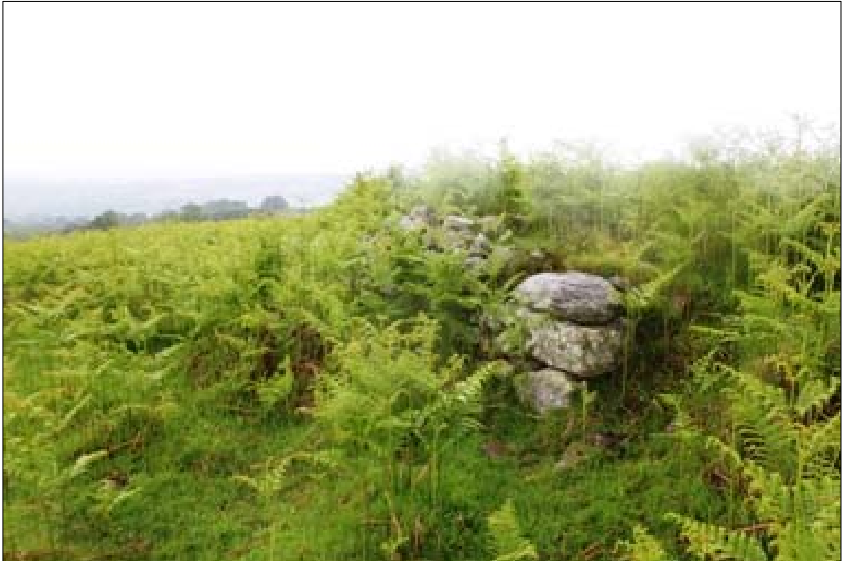
Figure 4a: Site 24; Wall at Boquhan Glen Farmstead from the Southeast with bracken
