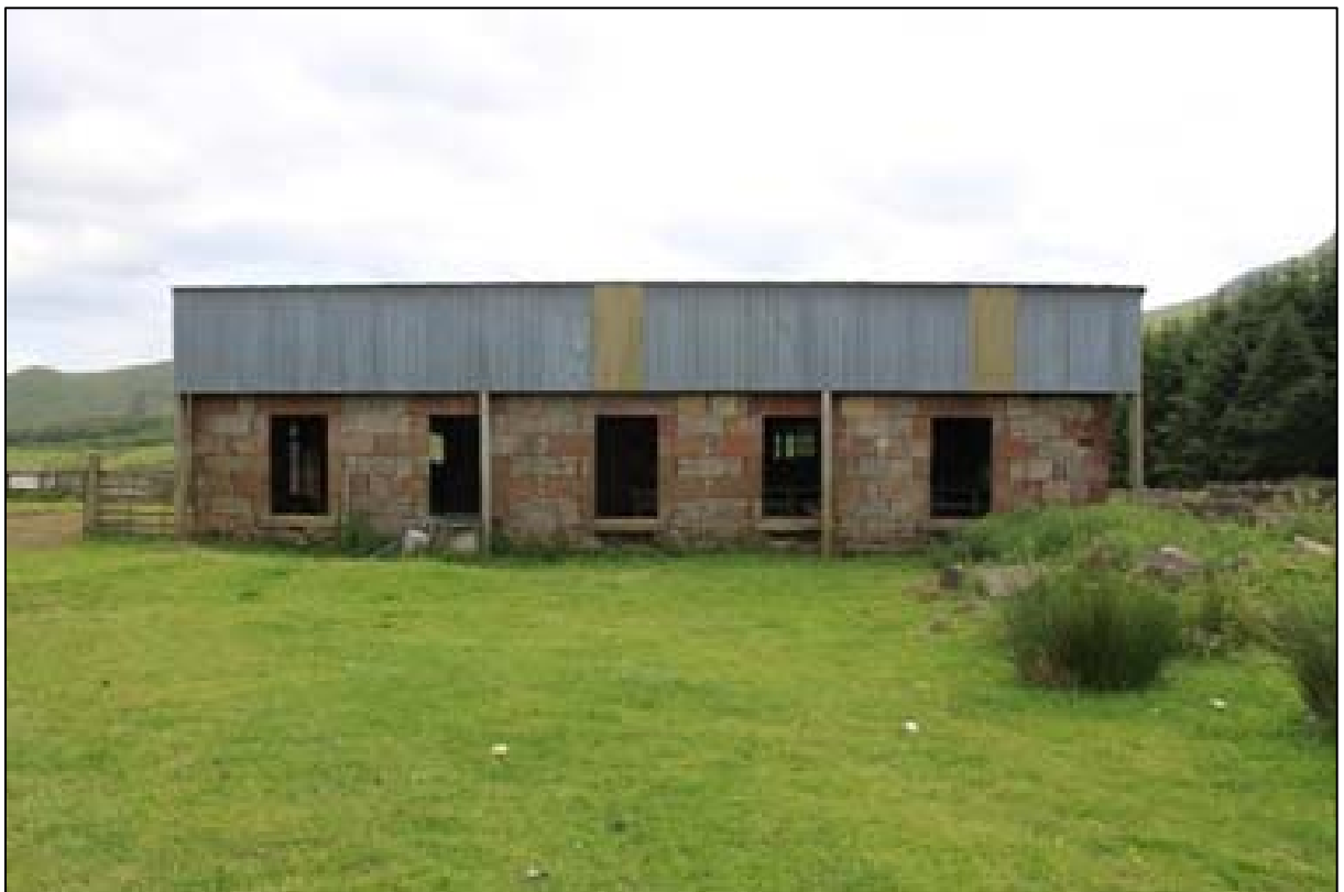
Figure 7b: Agricultural Building at Site 12 from the west.
