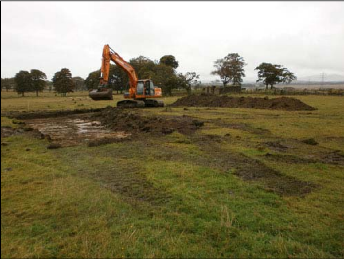
Figure 3a: Location shot, ground reduction (area of Crane Pads/Turbine base)
