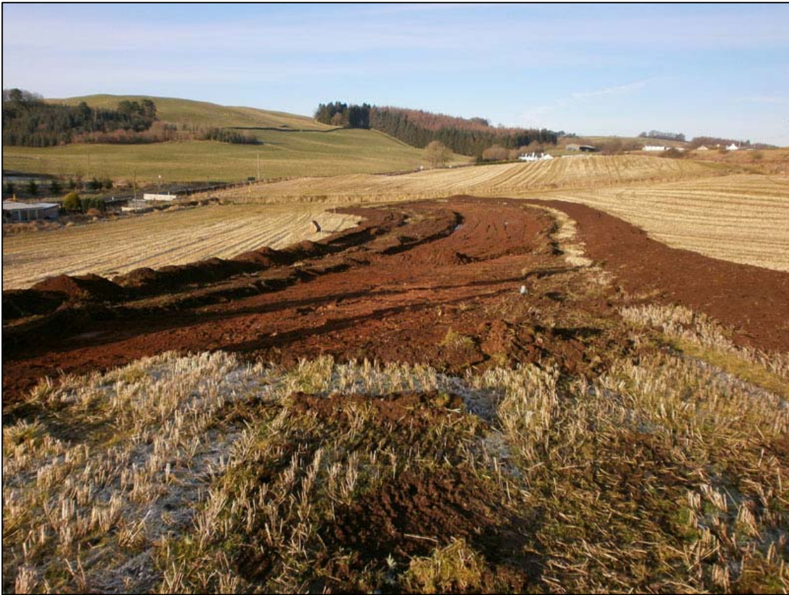
Figure 2a: Northern end of access road from the east-south-east
