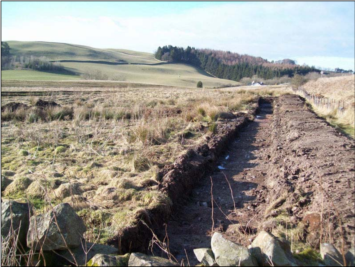
Figure 3a: Trenches in field to north of Scheduled Monument from the southeast
