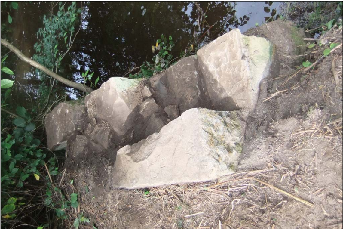
Figure 5b: Structural Remains [018] of pier
