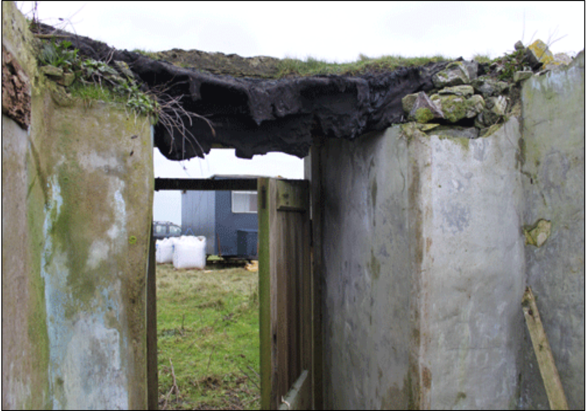
Figure 4a: Remnants of Black Felt Roof
