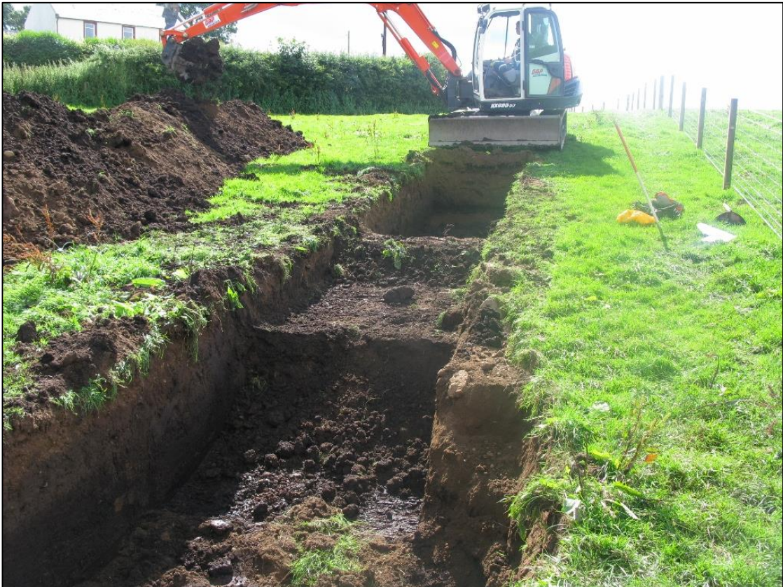
Figure 6b: General view of pinch-point 3 trench before abandonment, from the north-north-east.
