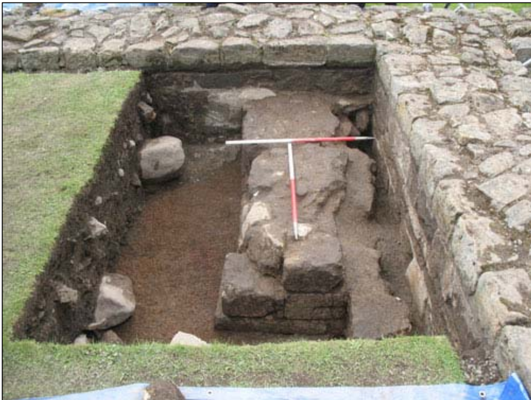
Figure 11b: Trench 15 looking west showing early wall
