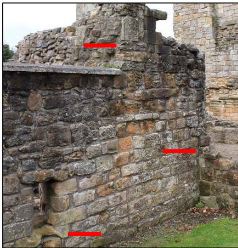
a: Three level of window cills
