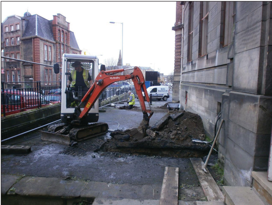
Figure 4b: Trench 1 being excavated
