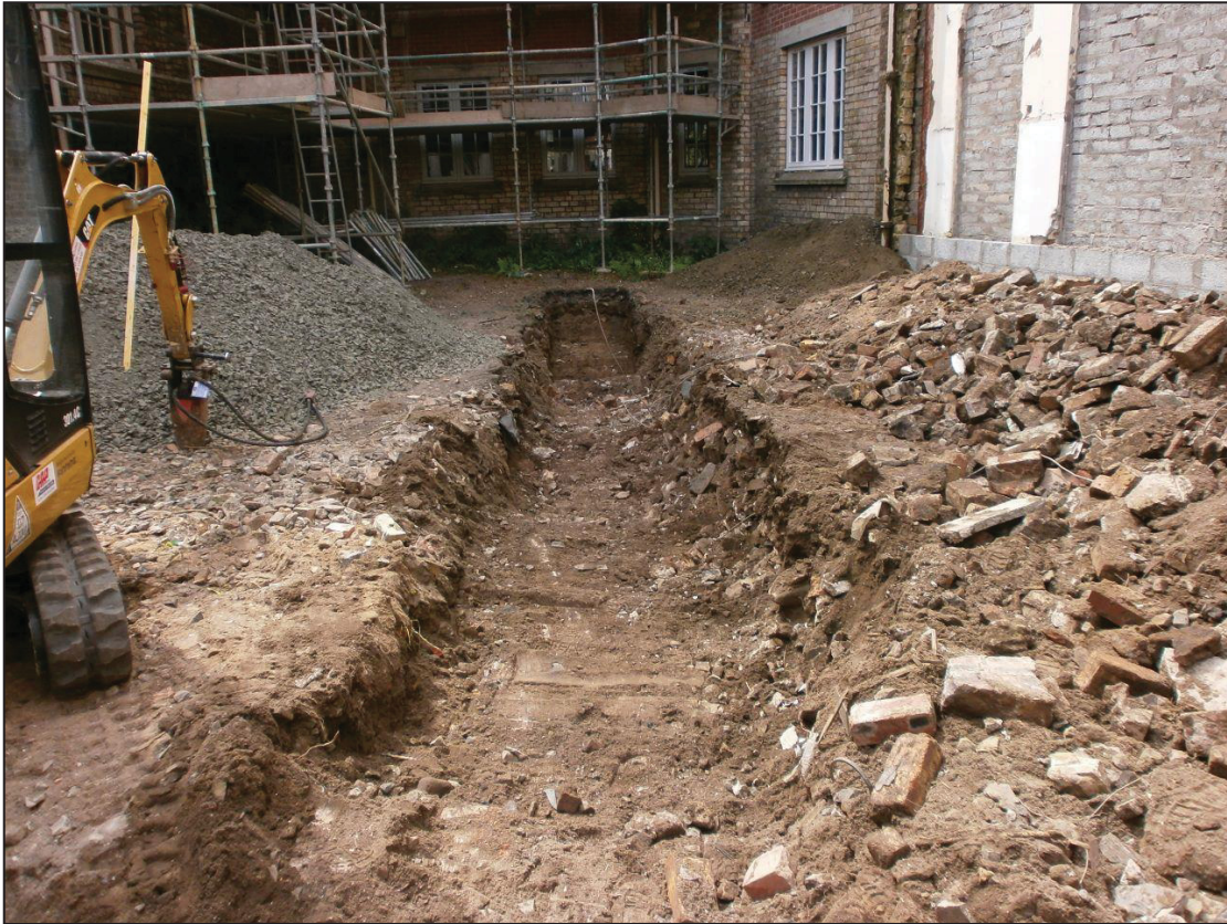
Figure 8a: Central Trench in the western courtyard
