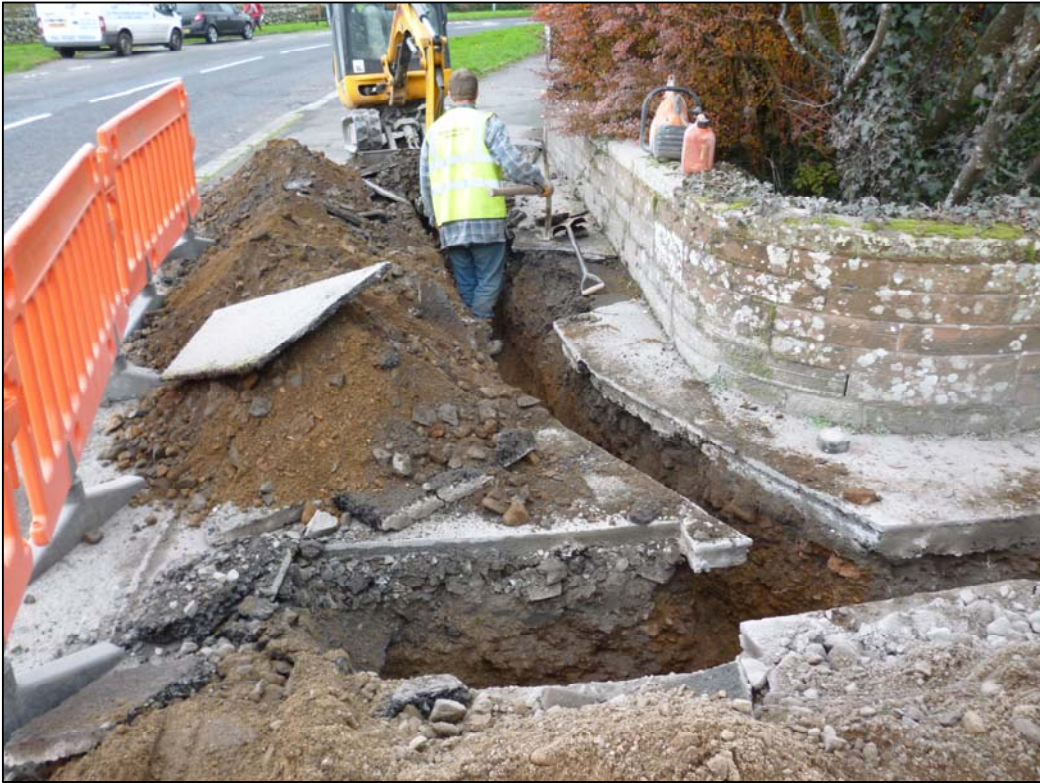
Figure 5a: Excavations on the pavement to connect water main
