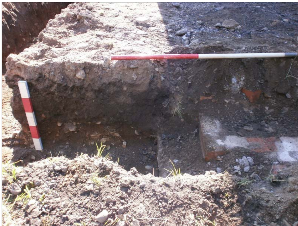
Figure 3b: West Facing Section of the foundation trench with [007] founds of previous extension.
