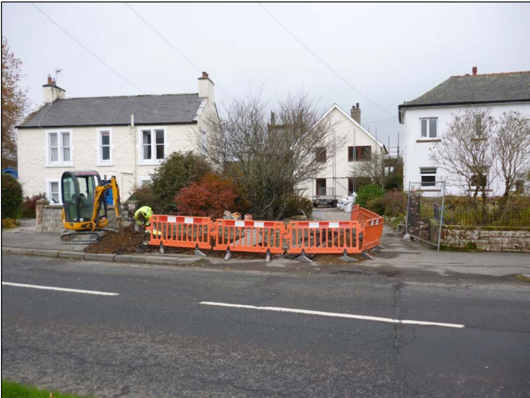
Figure 5b: Excavations on Main Street, New Abbey.
