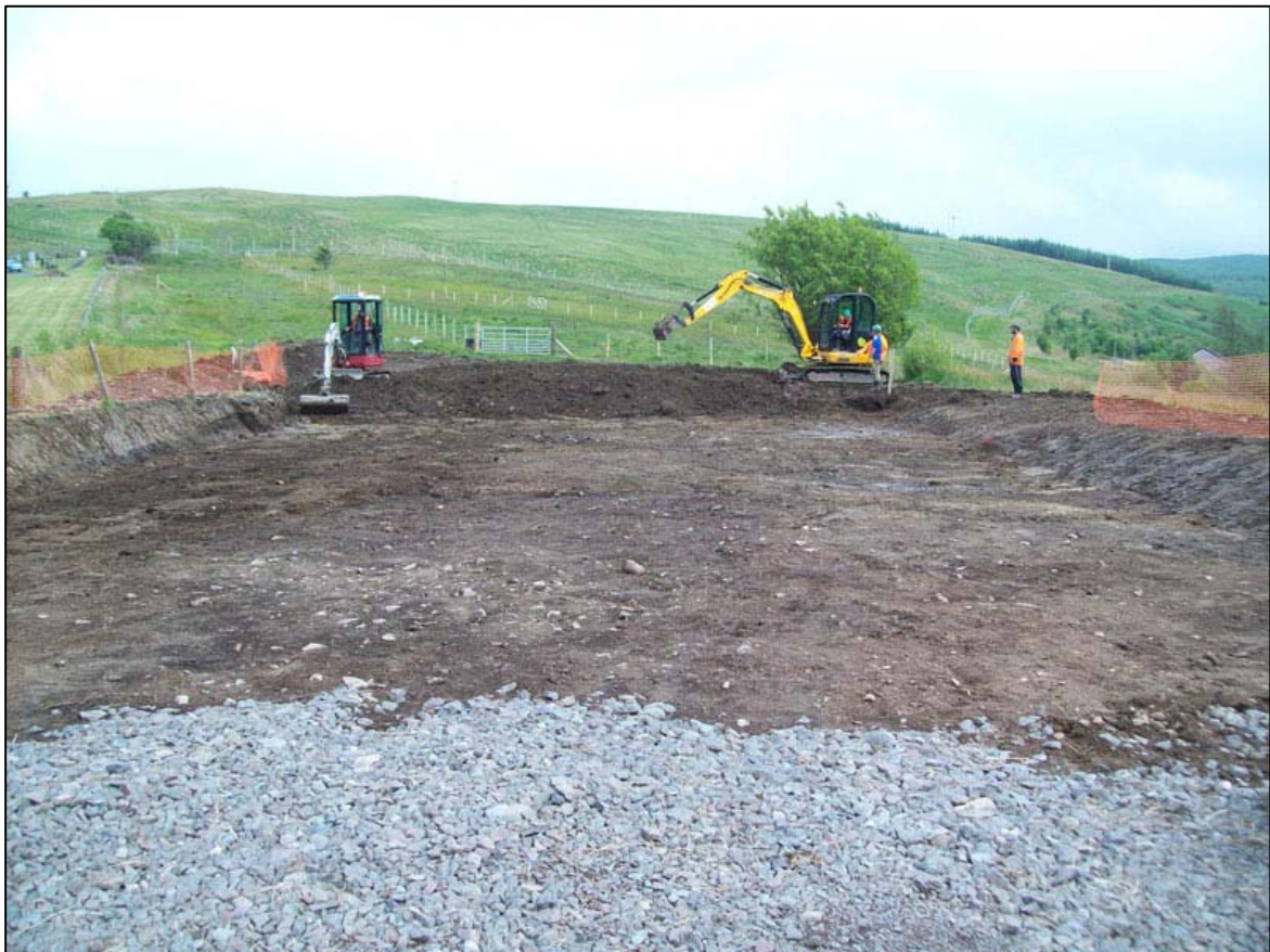
Figure 9b: Working shot – stripping the full carpark area from the west-north-west
