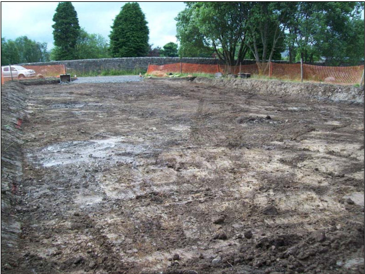
Figure 10b: Shot of carpark area fully excavated
