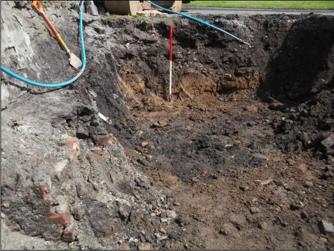
Figure 9: View of brick wall (003) abutting wall (010) and foundations of (010). From SW.
