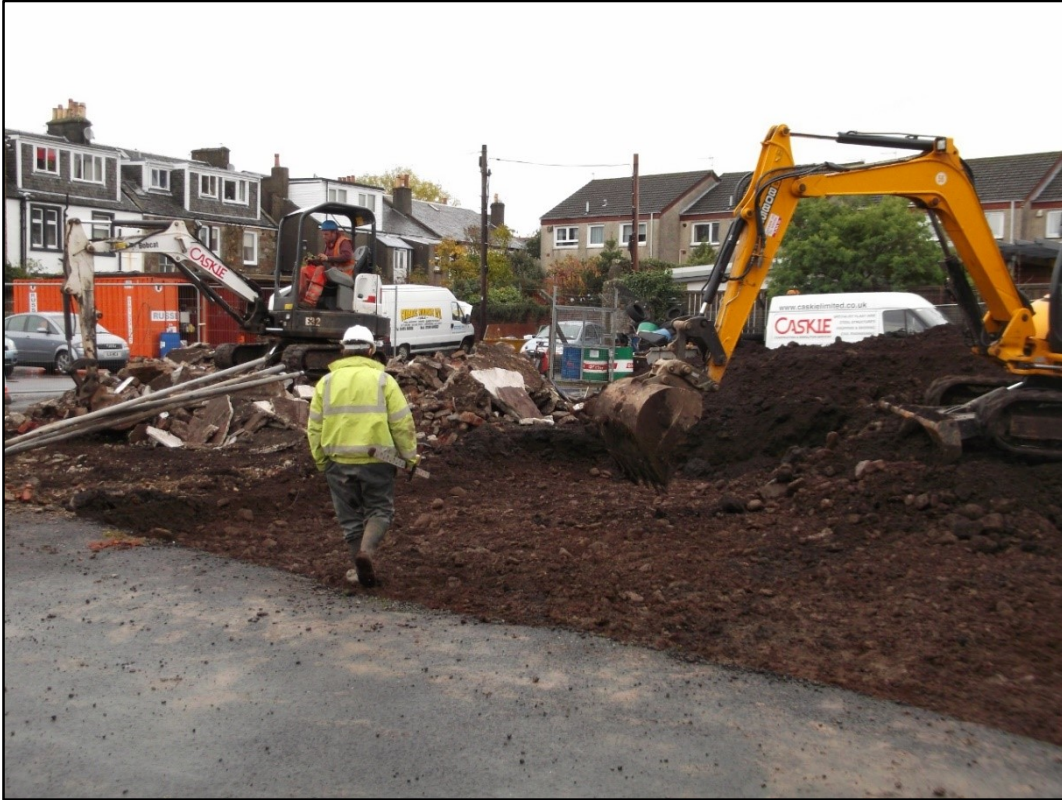
Figure 3a: Commencing works on reduction of ground level SW corner of site and removal of demolition debris in NW corner of site.
