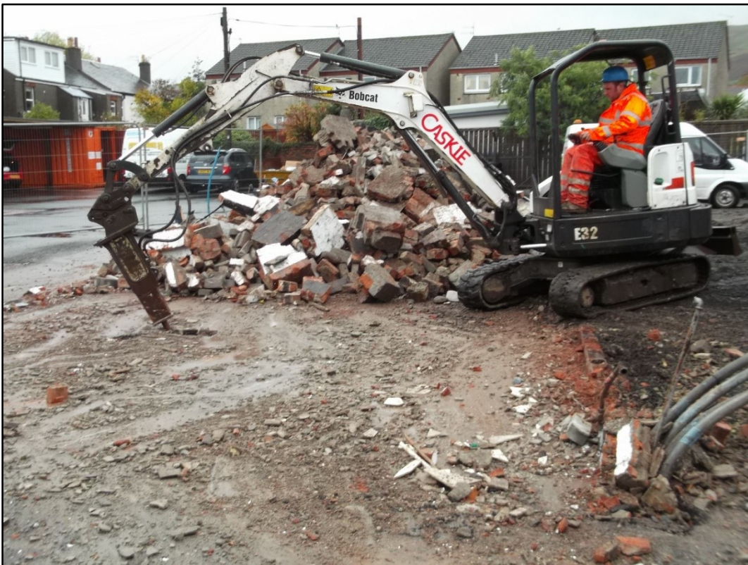
Figure 3b: Removal of concrete floor of demolished garage.
