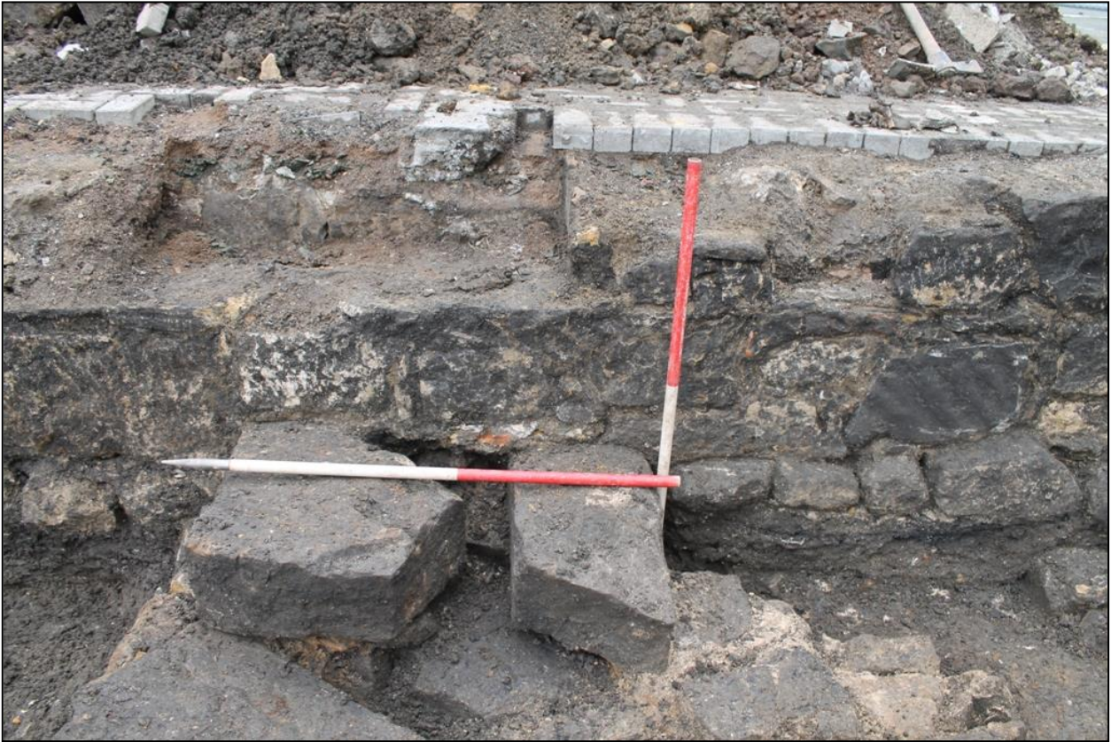
Figure 25a: Depicting the foundations of the present car park wall and re-use of stones from structure (115).
