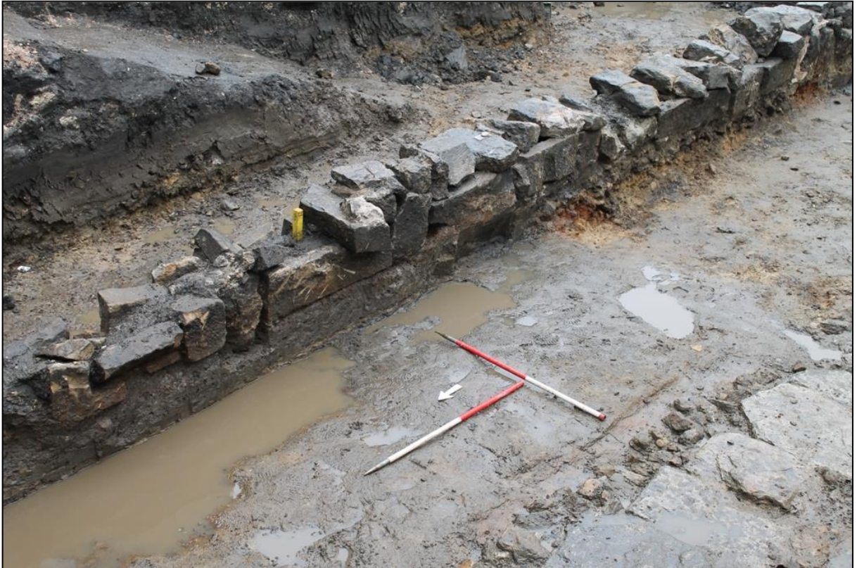
Figure 19a: West facing section of culvert (111).
