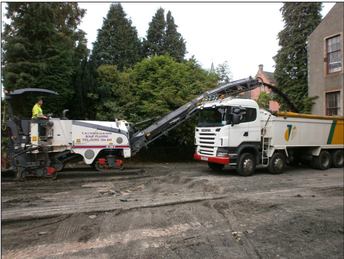
Figure 6b: Site preparation; planing and removal of the asphalt
