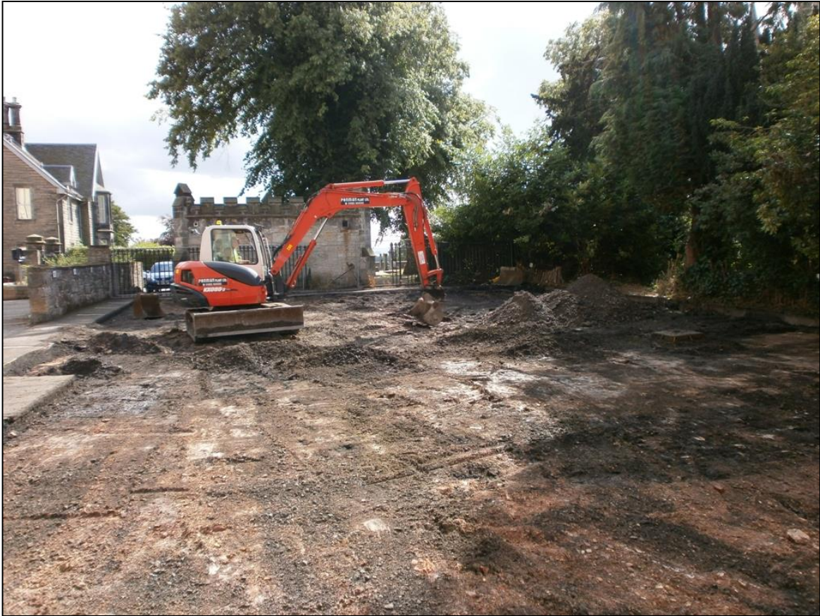
Figure 7a: Site preparation; removing modern overburden across the site
