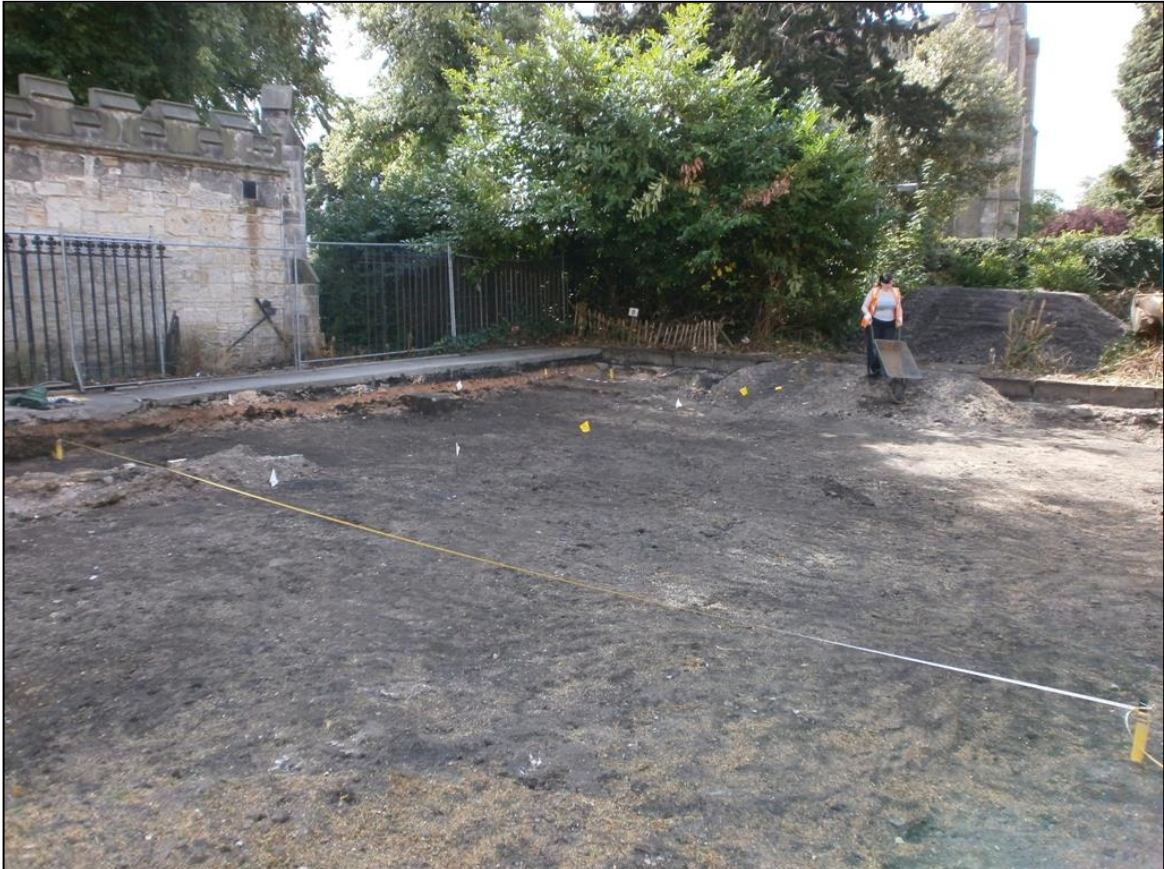
Figure 7b: Site preparation; site cleaning and flagging out areas for excavation
