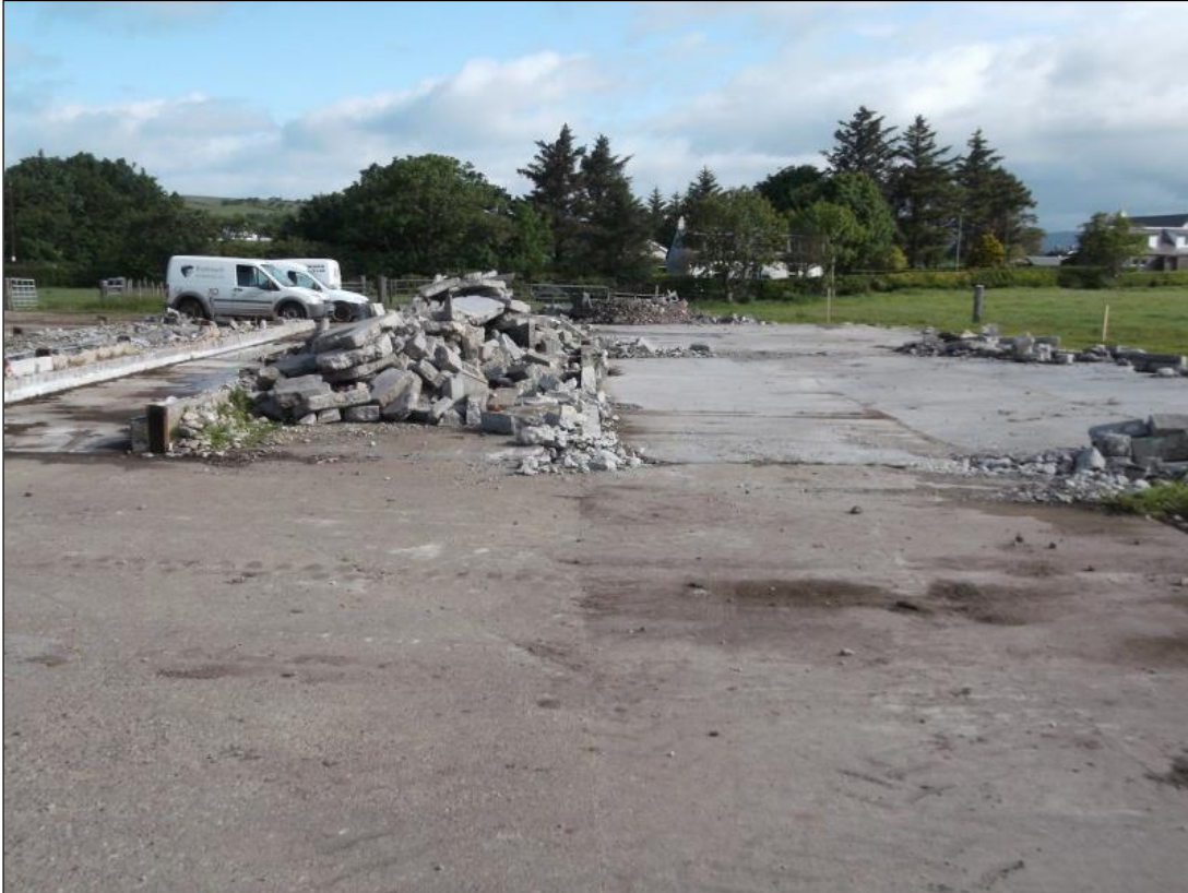
Figure 4: Pre excavation view of farmyard area. From southwest.
