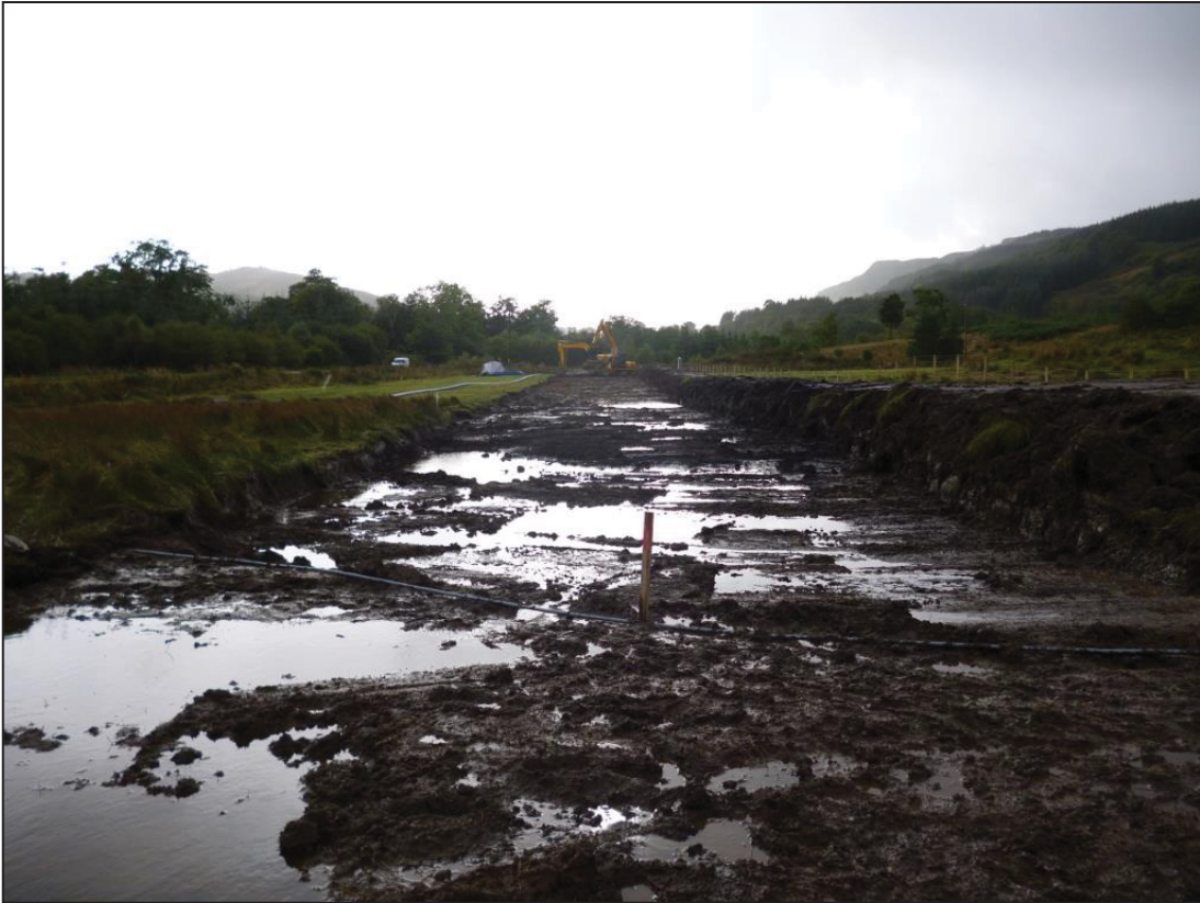
Figure 4a: Stripped section in Area C from the northeast
