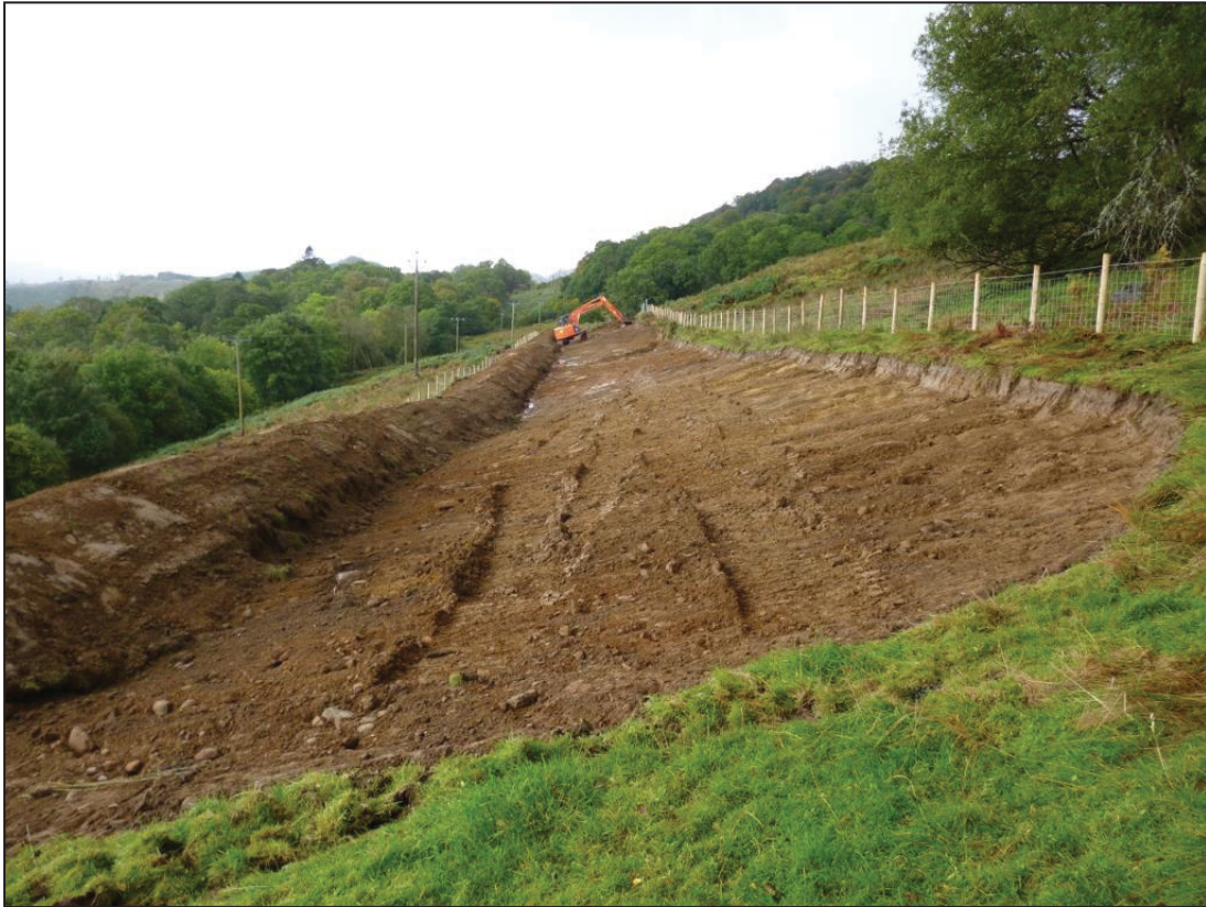
Figure 5a: Third section in Area H from the northeast
