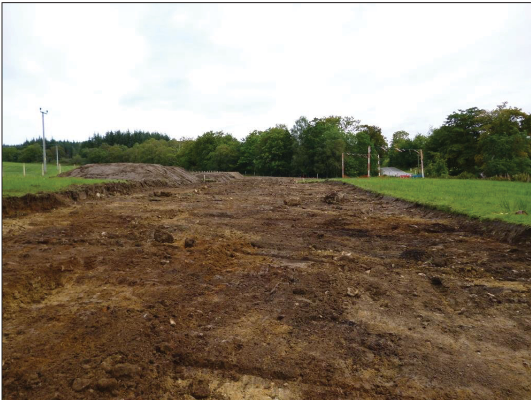
Figure 4b: General shot of Area D from the southwest
