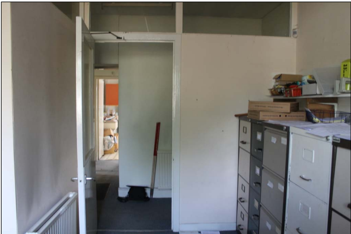
Figure 30b: Room C, W wall taken from the E.
