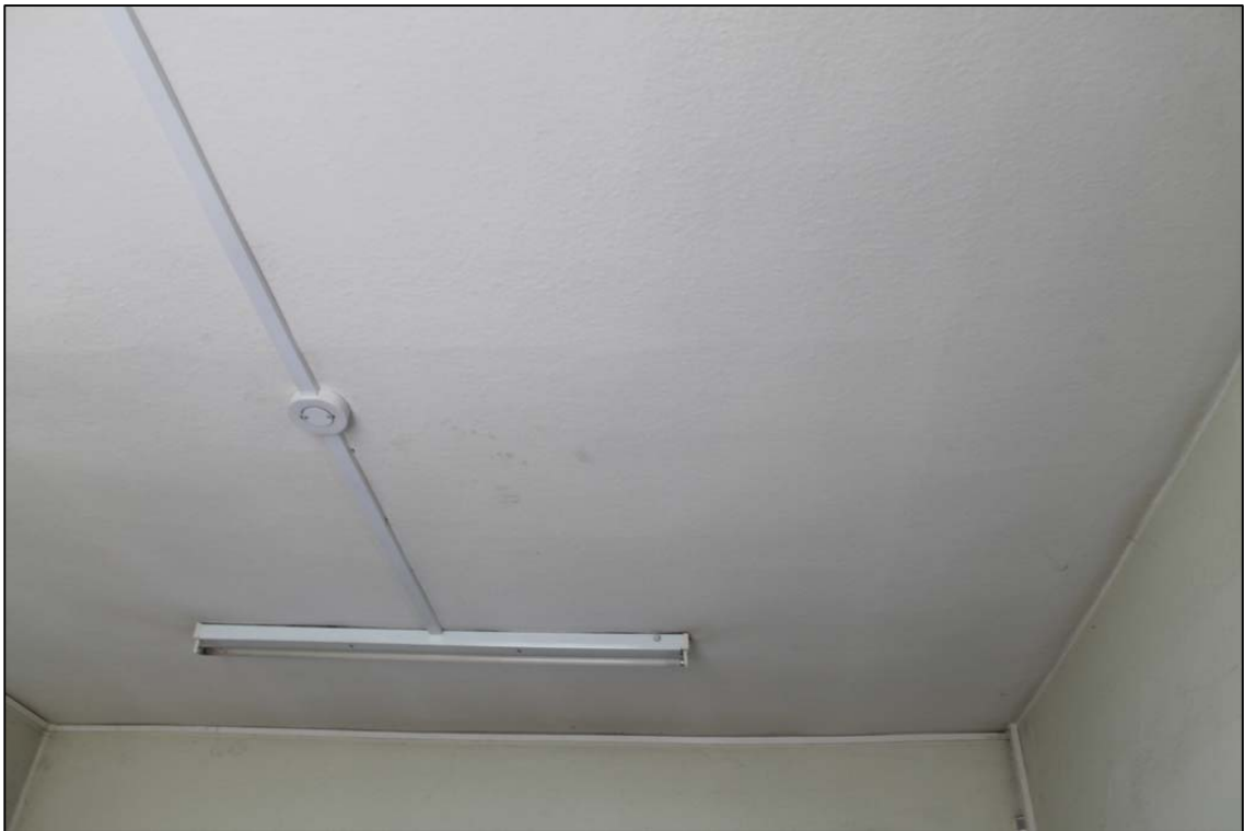
Figure 19b: Room A (ground floor), ceiling taken from the E
