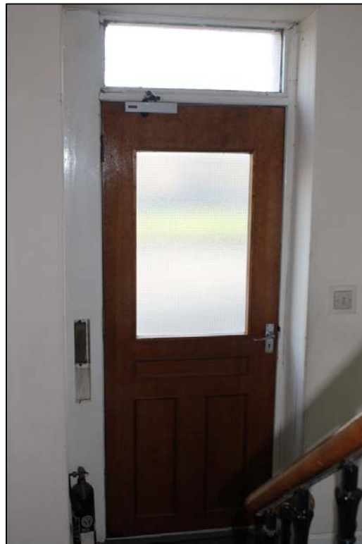
Figure 24b: Stairway/hallway (ground floor), main access door taken from N.
