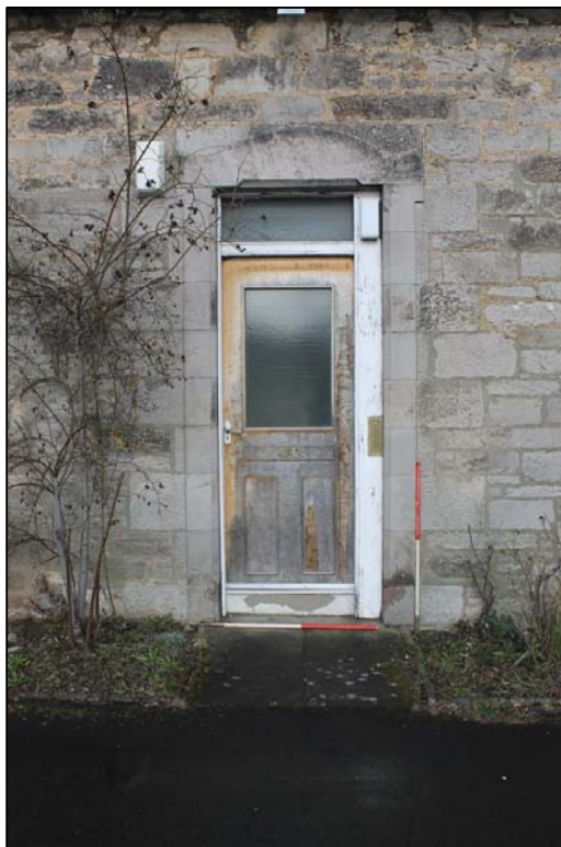
Figure 8b: Detail of main access on N elevation taken from S.
