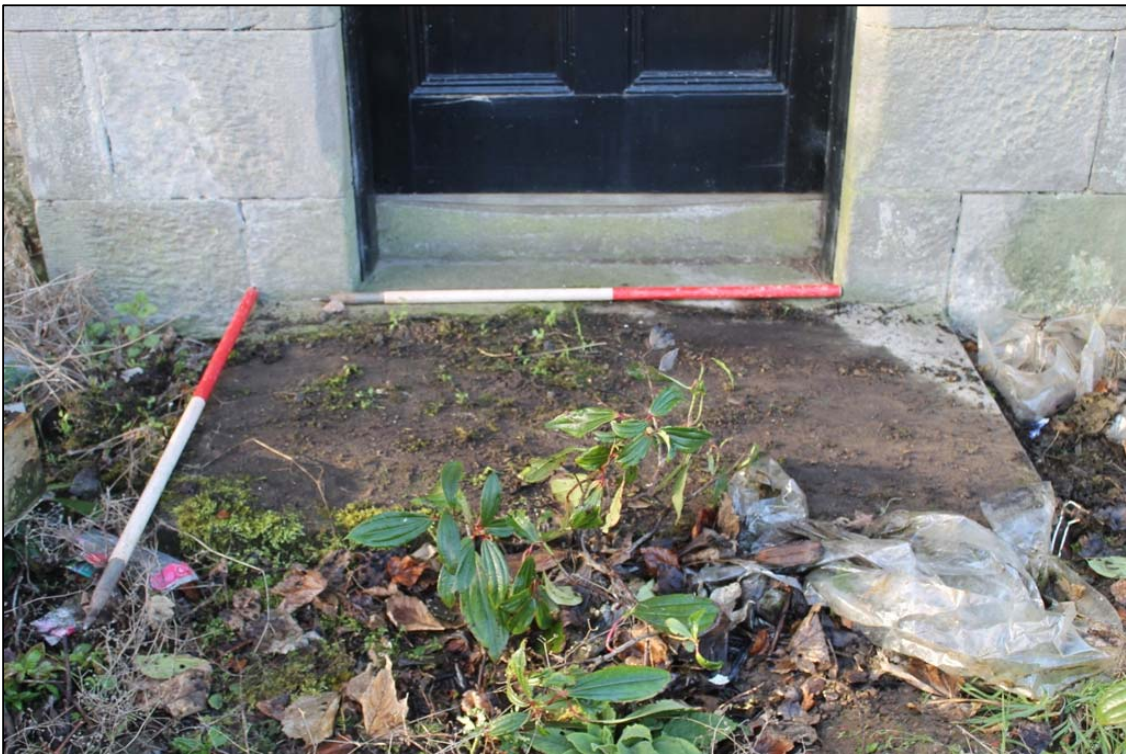
Figure 10b: Detail of flagstone/threshold on W elevation taken from E.
