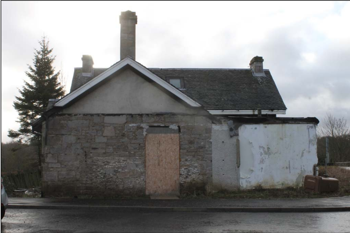
Figure 11a: S elevation of Building B and modern extension taken from the N.
