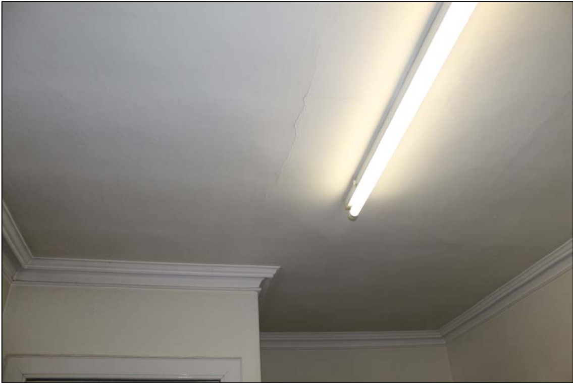
Figure 33: Room D, ceiling and cornices taken from N.
