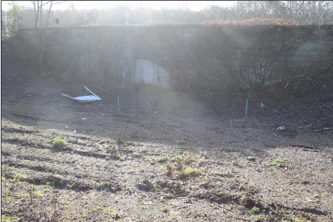
Figure 13b: S elevation of railway bridge taken from the NW.
