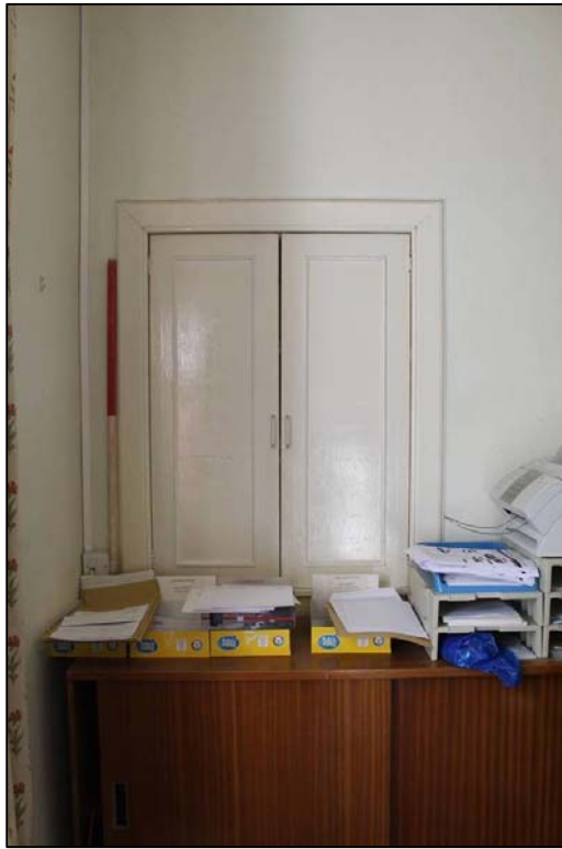
Figure 19a: Room A (ground floor), Alcove on W wall taken from the E.
