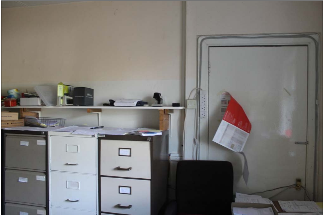
Figure 30a: Room C, N wall and porch access taken from the S.
