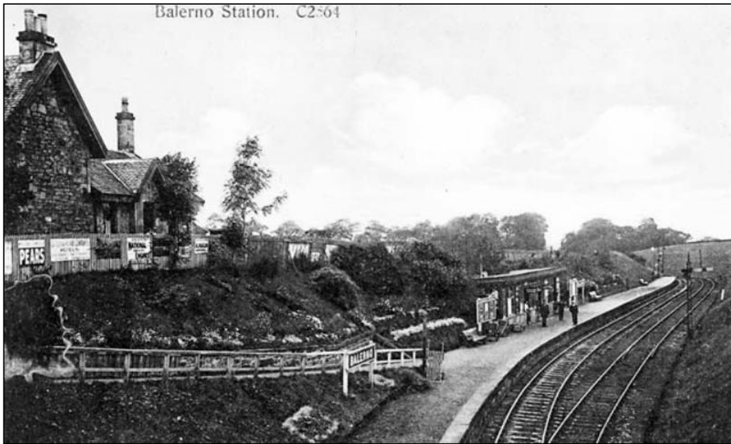
Figure 3a: Photo of Balerno Station taken c1910 illustrating the location of the platform and railway line with the Station Office visible to the left of the photo (www.edinphoto.org.uk 20/02/2014).
