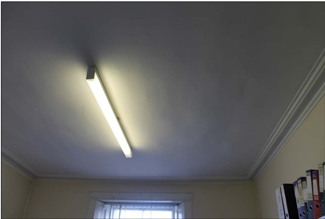
Figure 22: Room B (ground floor), ceiling taken from N.
