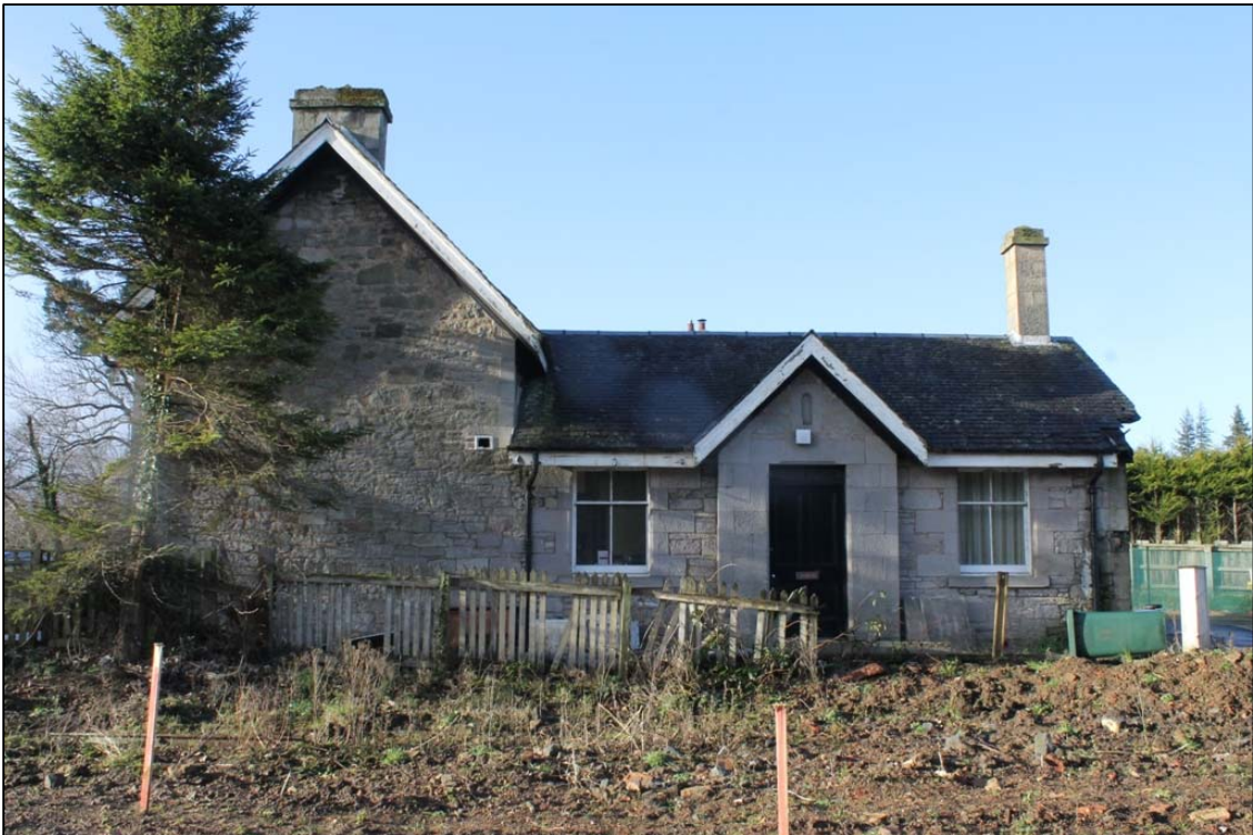
Figure 7b: W elevation of Buildings A and B taken from the E.
