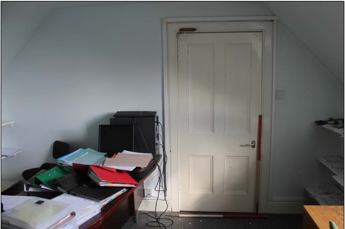
Figure 36b: 1 st floor Room A, E wall and doorway taken from W.
