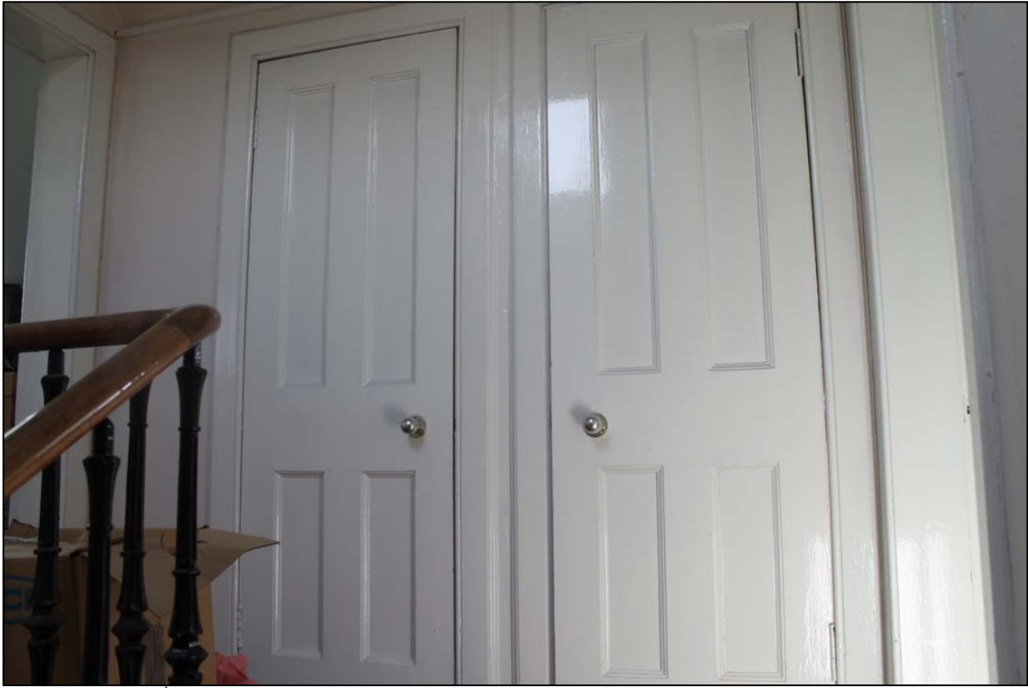
Figure 39a: 1 st floor landing, S wall and cupboards taken from N
