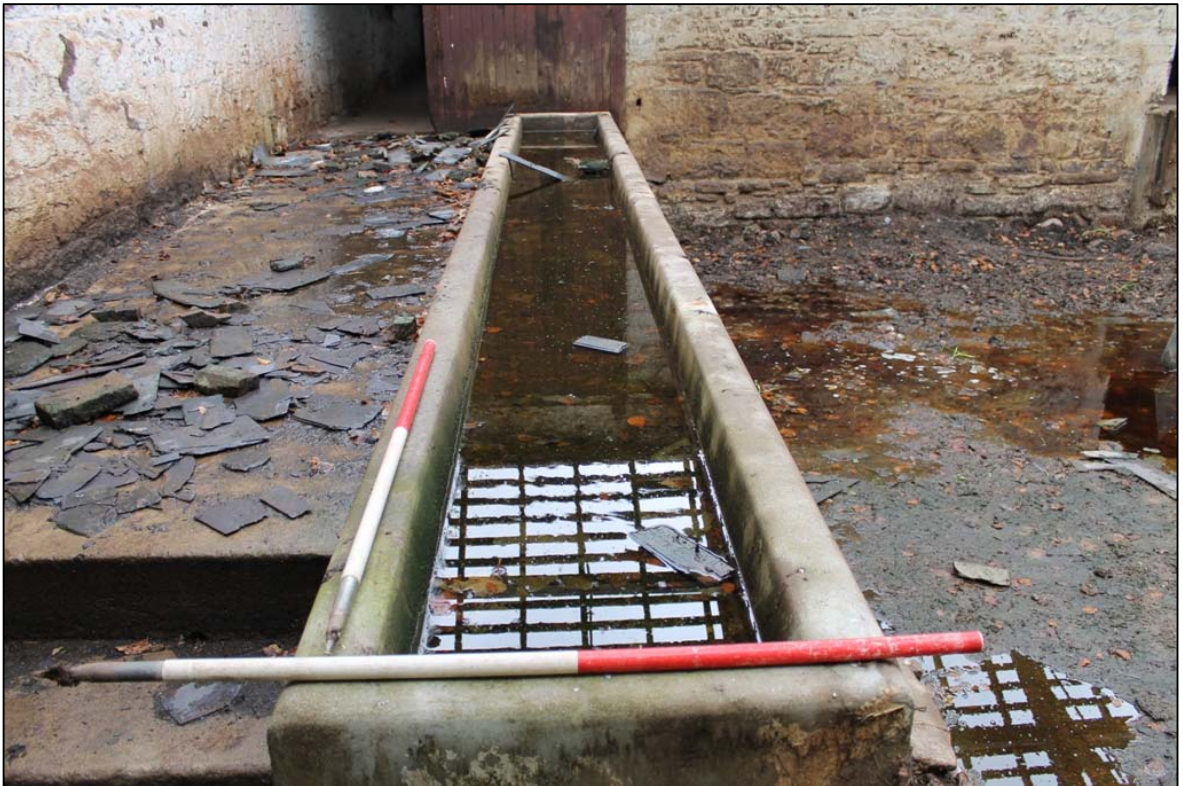
Figure 13b: Water/food trough I at the north end of Room C
