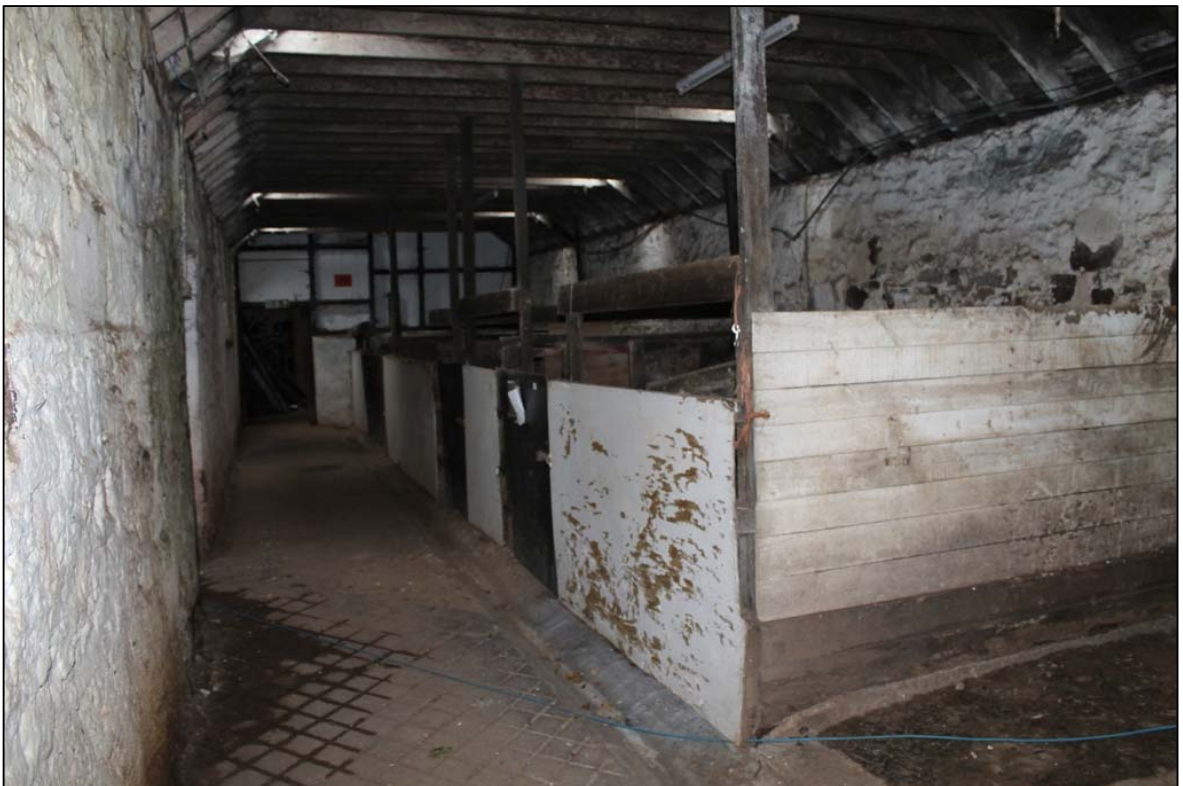
Figure 16b: Room G looking west and showing the animal pens
