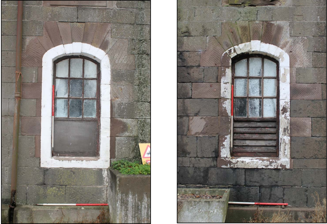
Figure 6a: Windows 2 (i) & (ii) in the southern wing/elevation
