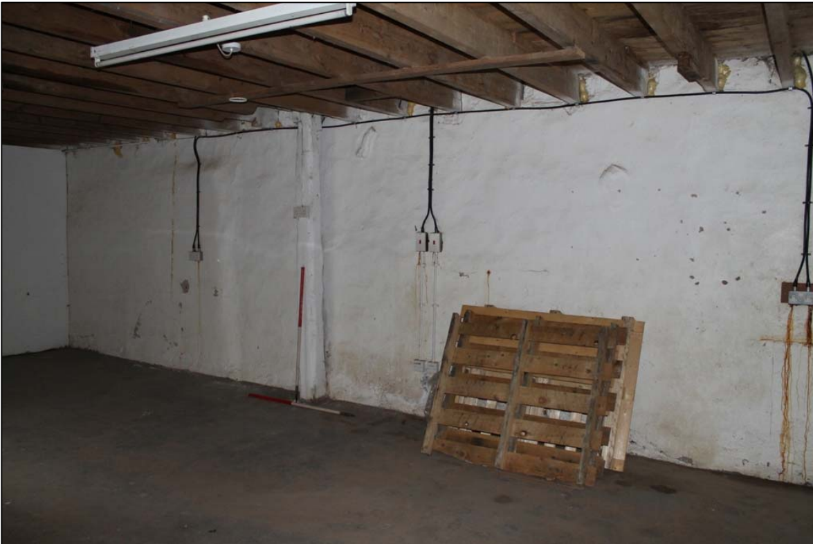
Figure 12b: Room B east wall illustrating the white wash render, floor, ceiling and modern fixtures
