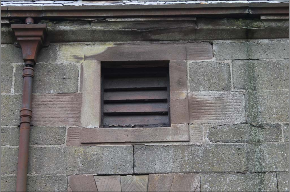
Figure 7a: Second storey window/air vent 4 (i)
