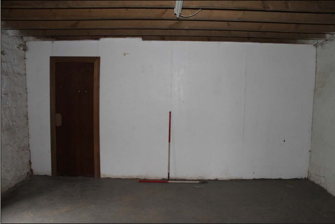
Figure 12a: Room B illustrating the partition, floor and ceiling
