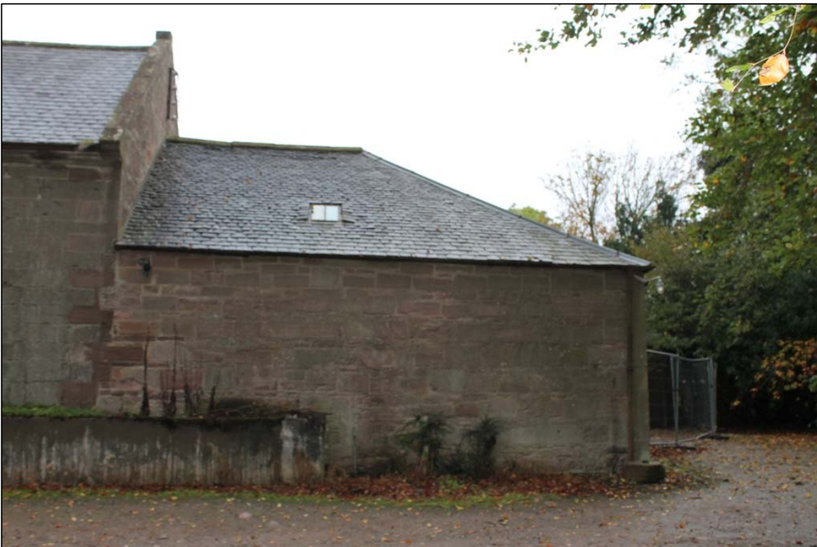
Figure 5b: Southern wing east end extension
