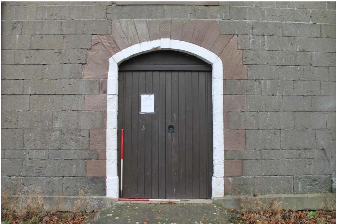
Figure 6b: The centrally located segmentally arched doorway 3(i)
