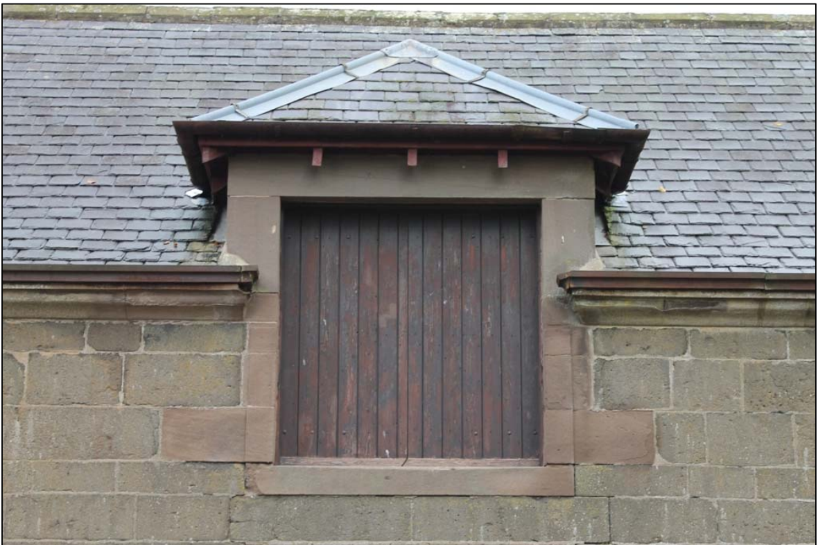
Figure 7b: The centrally located second storey access (5)
