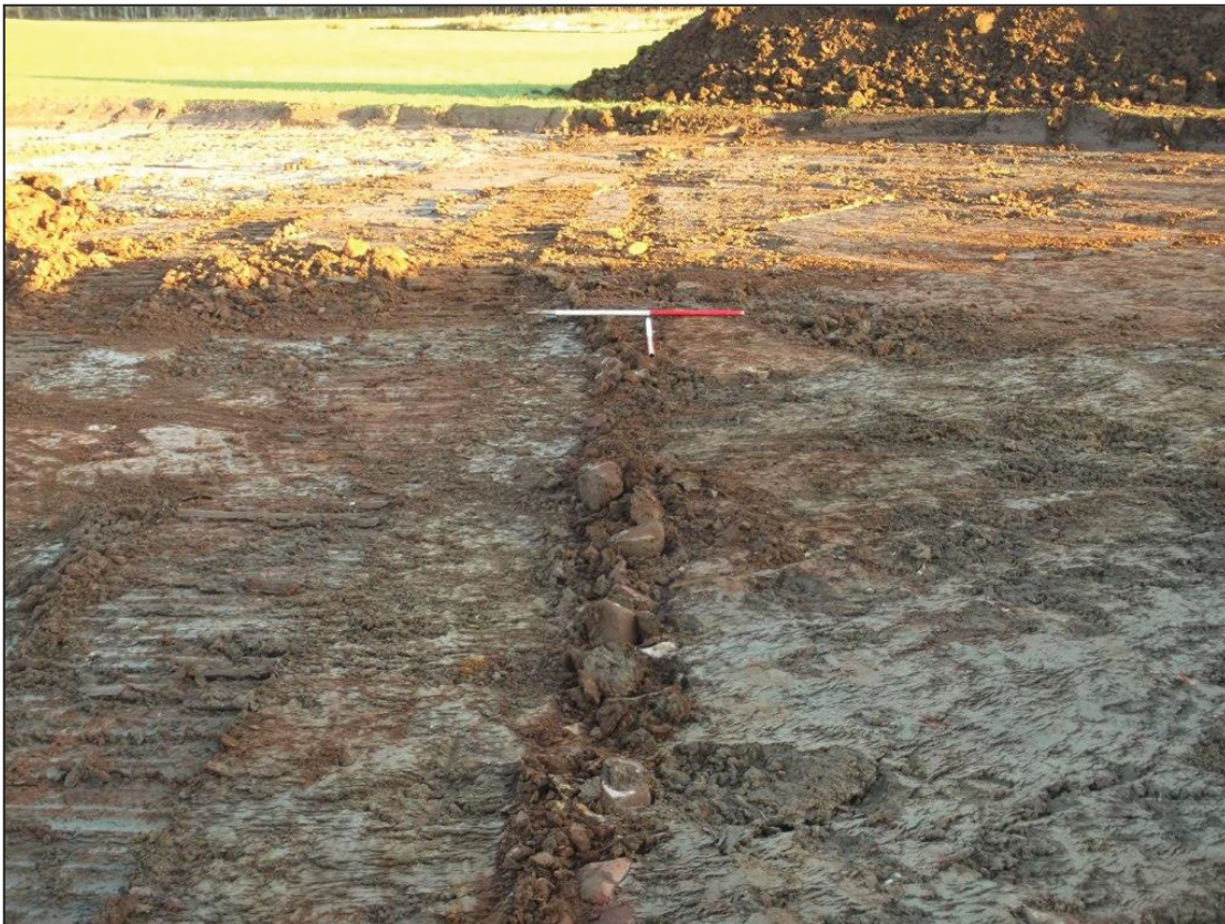
Figure 14b: Rubble/French drain.
