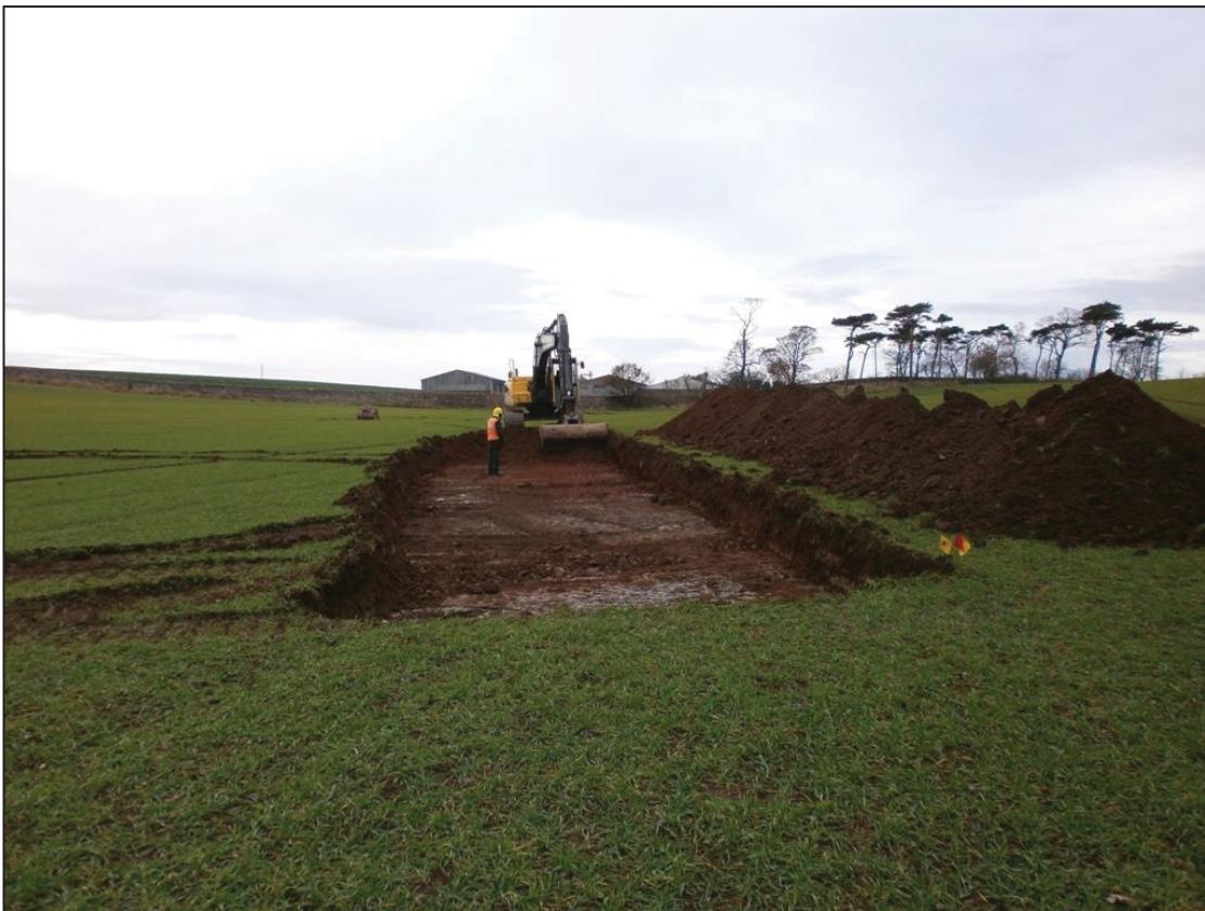
Figure 6b: Showing the commencement of the monitored topsoil strip
