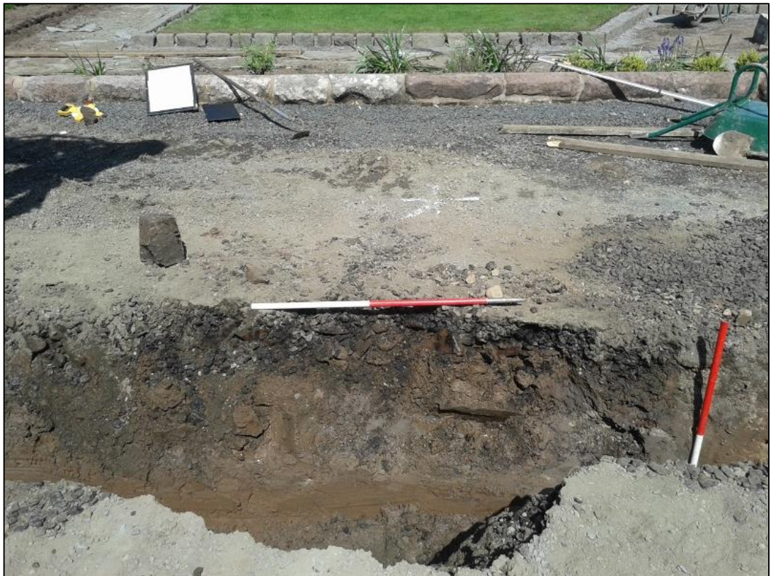
Figure 11: South facing section at western end of T4 showing stone foundation [008].
