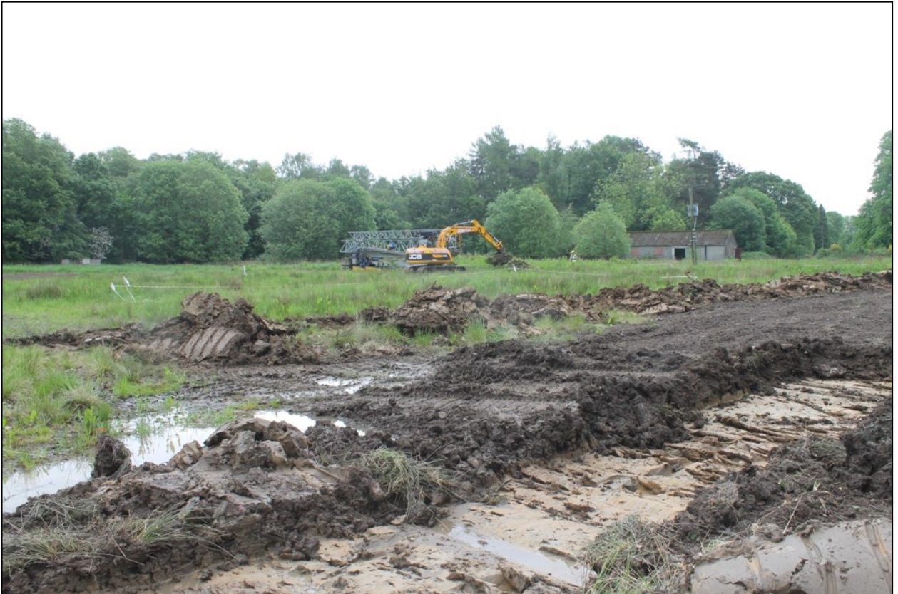
Figure 5a: Depicting the development site with the vegetation cover and clay subsoil with waterlogging in areas.
