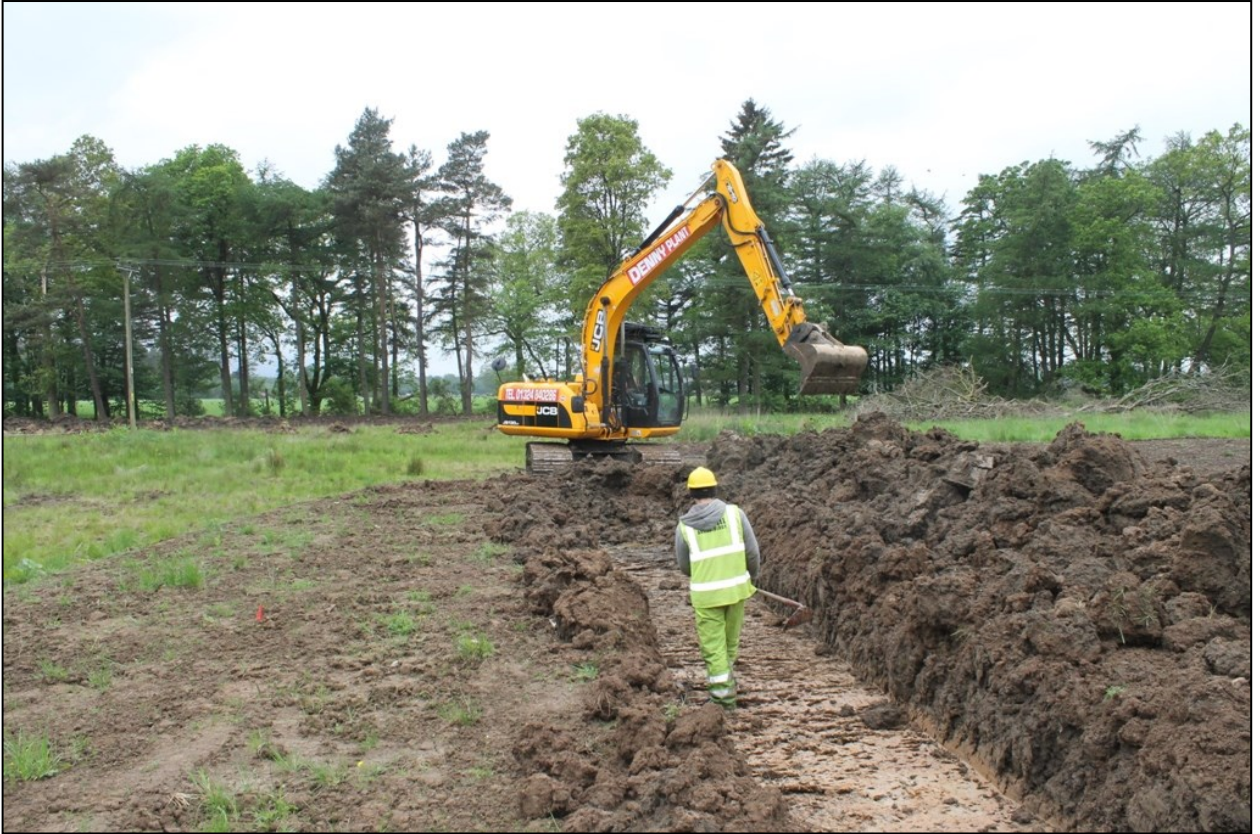
Figure 4a: Excavating trenches.
