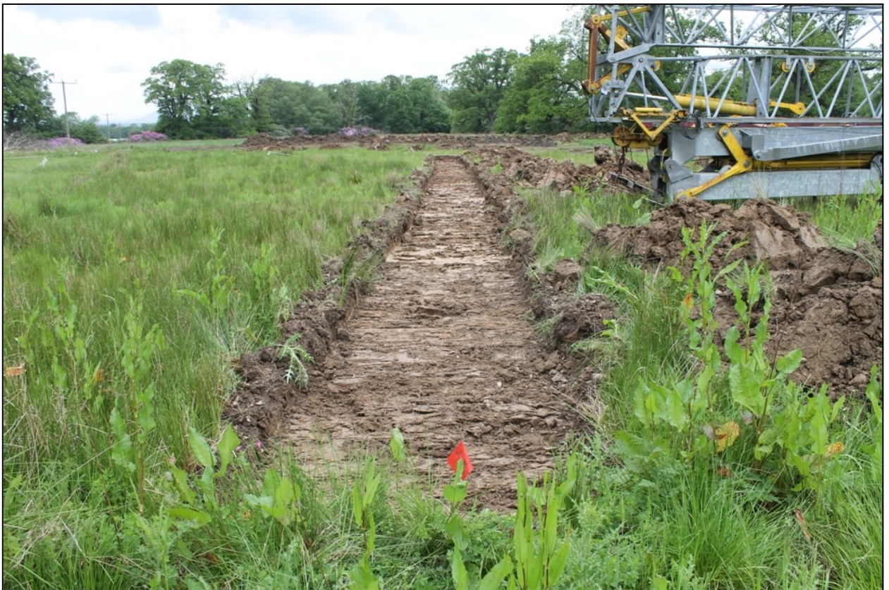
Figure 6b: Trench 6 demonstrating subsoil (004).
