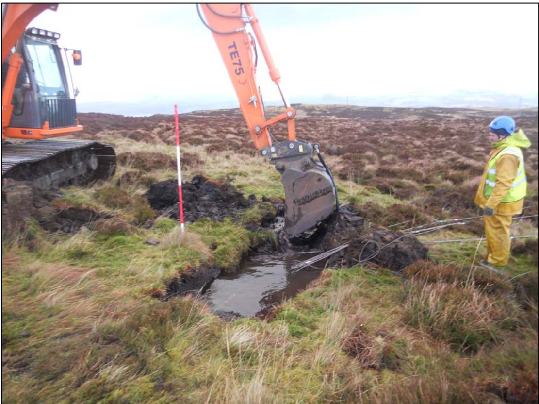
Figure 6: Drainage from A4
