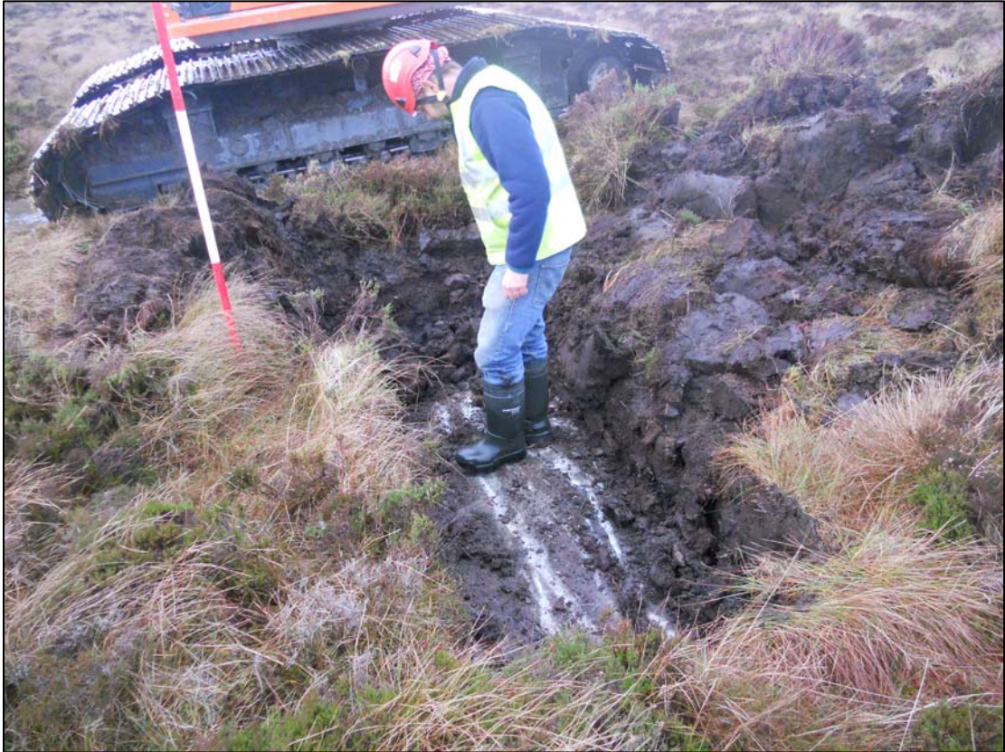
Figure 3: A1 excavated to bedrock
