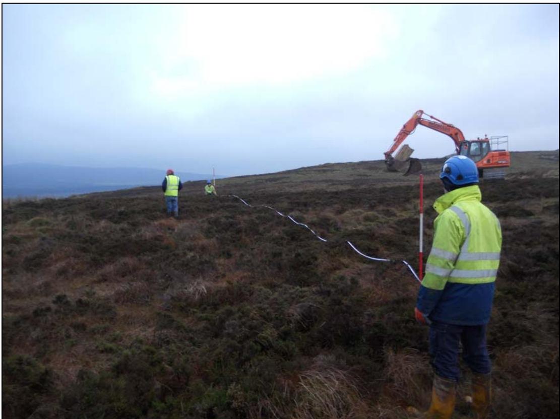
Figure 2: Laying out the Anchor Points
