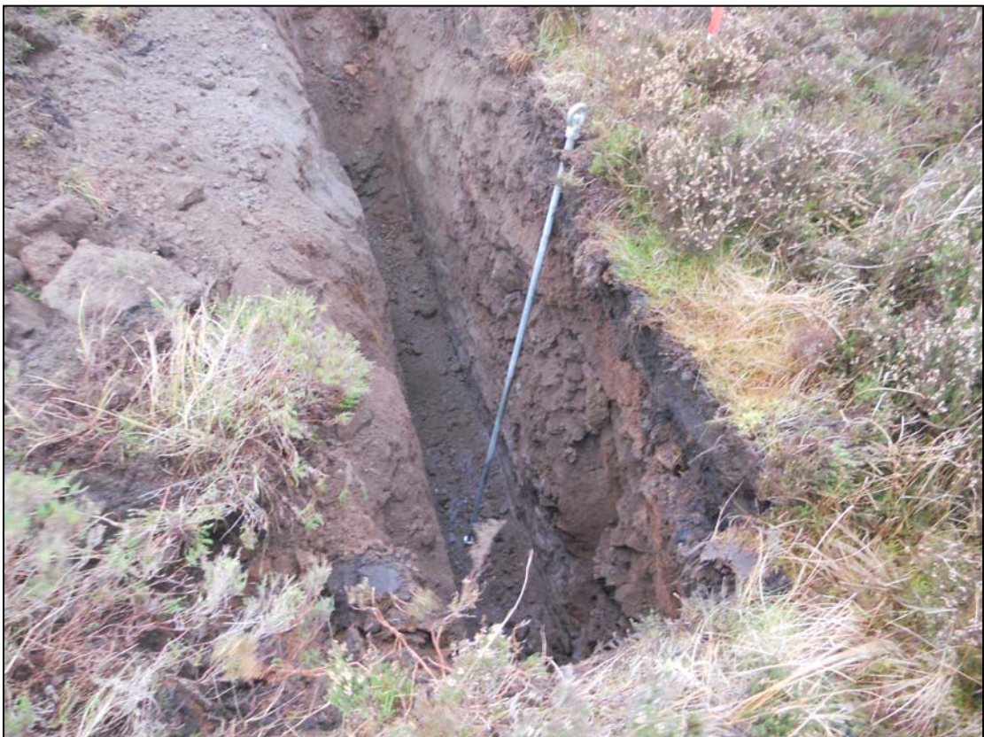
Figure 4: A5 excavated to 2m depth
