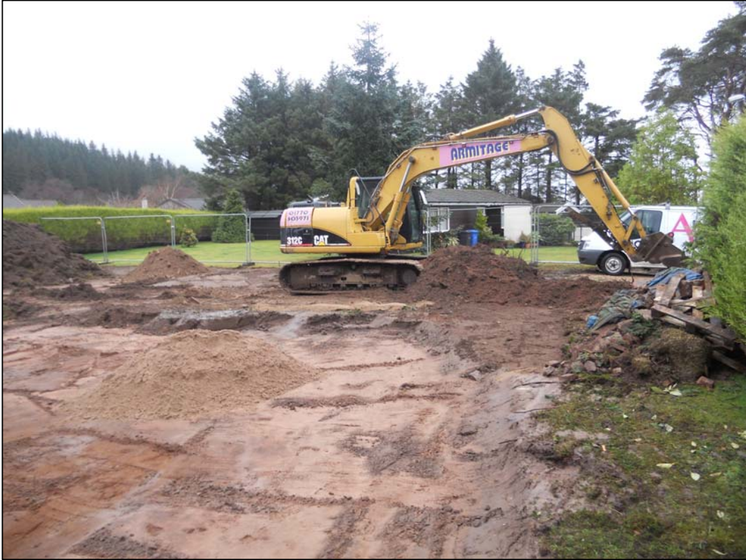
Figure 3a: Preparing to strip the north-eastern third of the site
