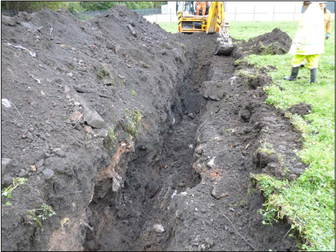
Figure 2: Trench 2 from the south
