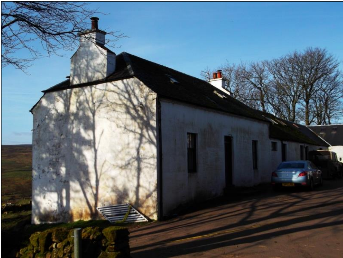
Figure 3a: View showing north elevation of farmhouse, pre-demolition
