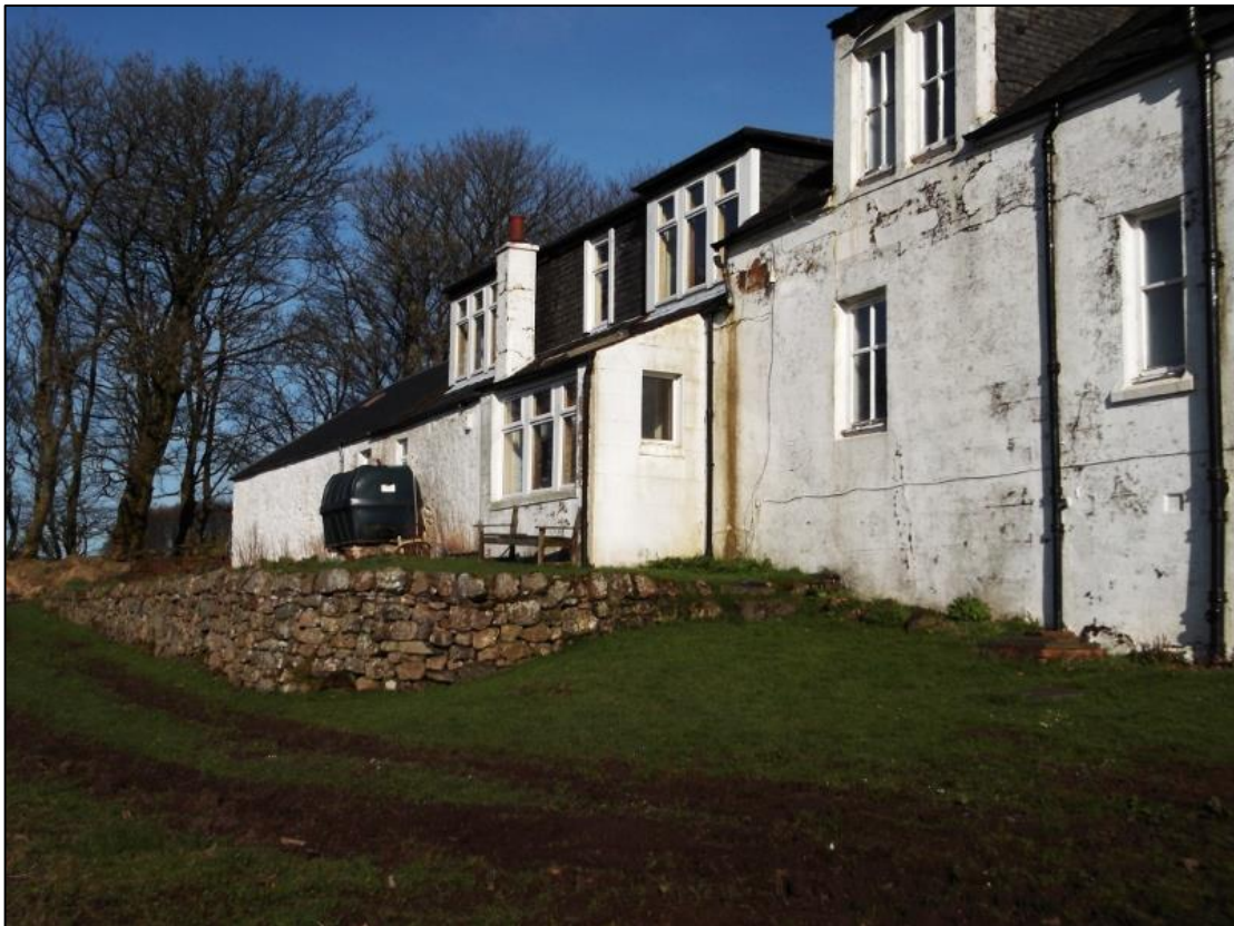
Figure 3b: Rear of farmhouse, with revetment wall forming garden terrace
