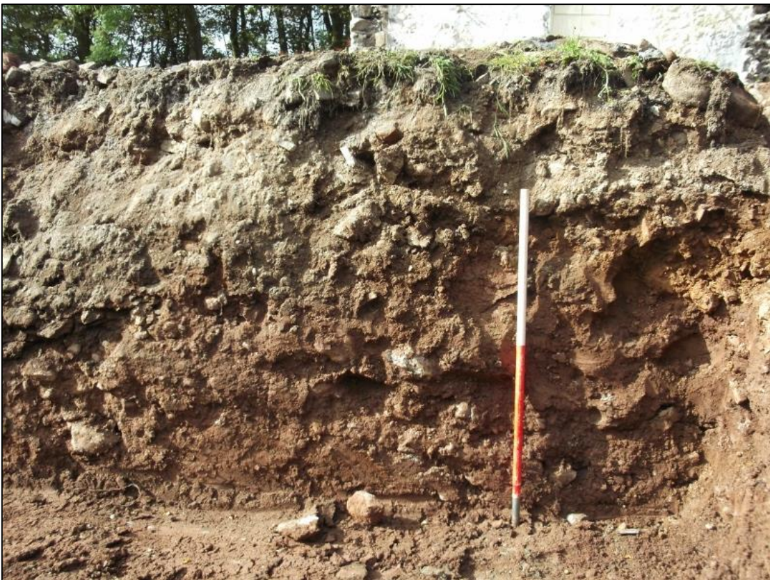
Figure 6b: Soil profile across NNW-SSE axis of site ('Trench c '), showing gravel mound (106) and made ground (105)
