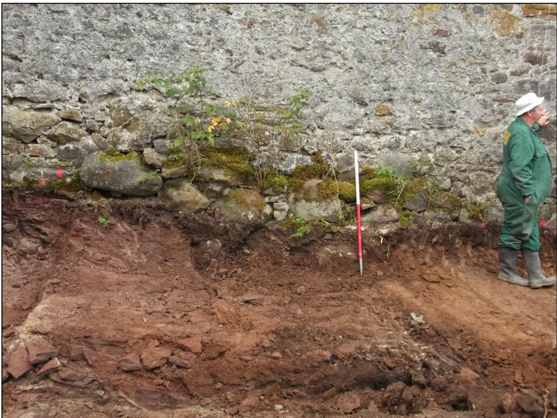
Figure 6b: Post-Excavation View of SW Gable Wall, revealing Bedrock (202) and Deposit (204) Underlying Base of Wall
