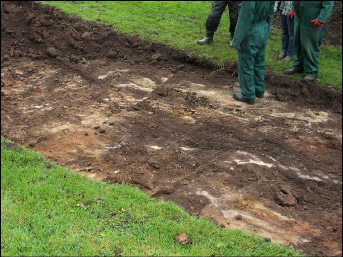
Figure 5a: Access Road, W End: Bedrock (102) with remains of Metalled Layer (103) overlying
