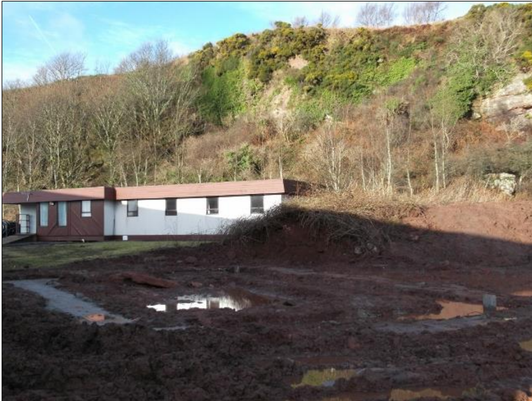
Figure 3a: Post excavation view of building 2 and the surrounding area. From the ESE
