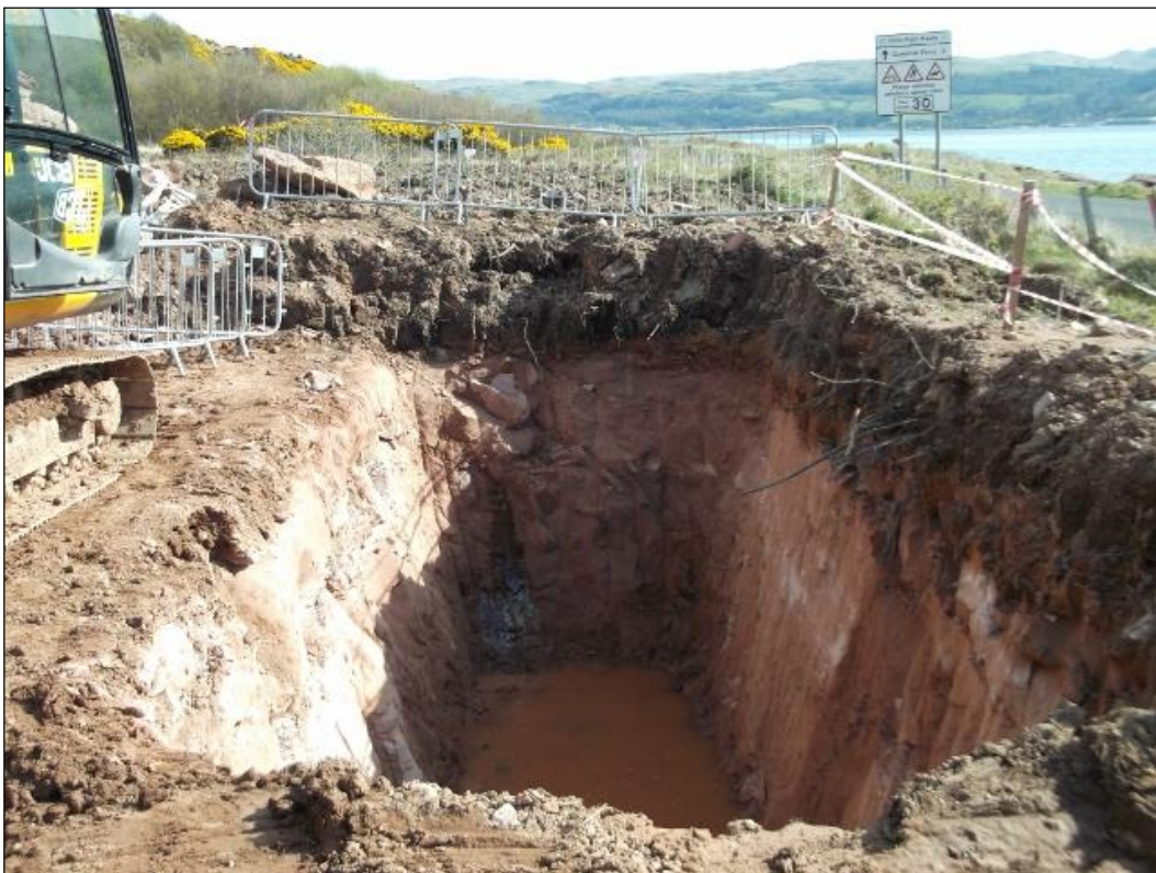
Figure 4b: Post excavation view of septic tank pit. From SW.
