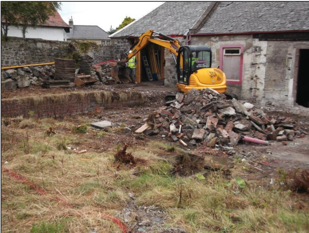
Figure 3b: Pre-excitation view from S, showing NE end of extant mid-19 th century cottage and late 19 th century extension
