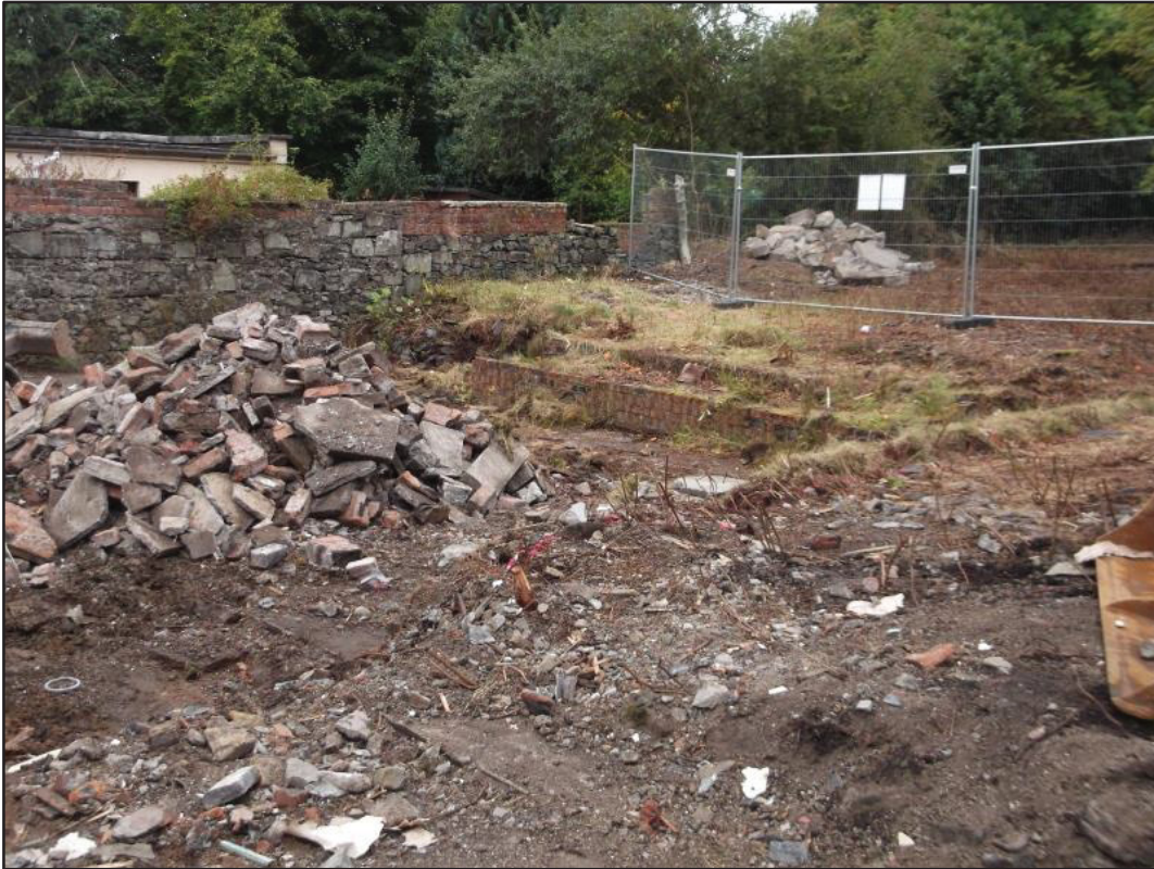
Figure 5a: Looking S across garden plot to rear of cottage, towards (from l to r), SE boundary wall, drystone revetment wall (004) and late 20 th century brick revetted terraces.
