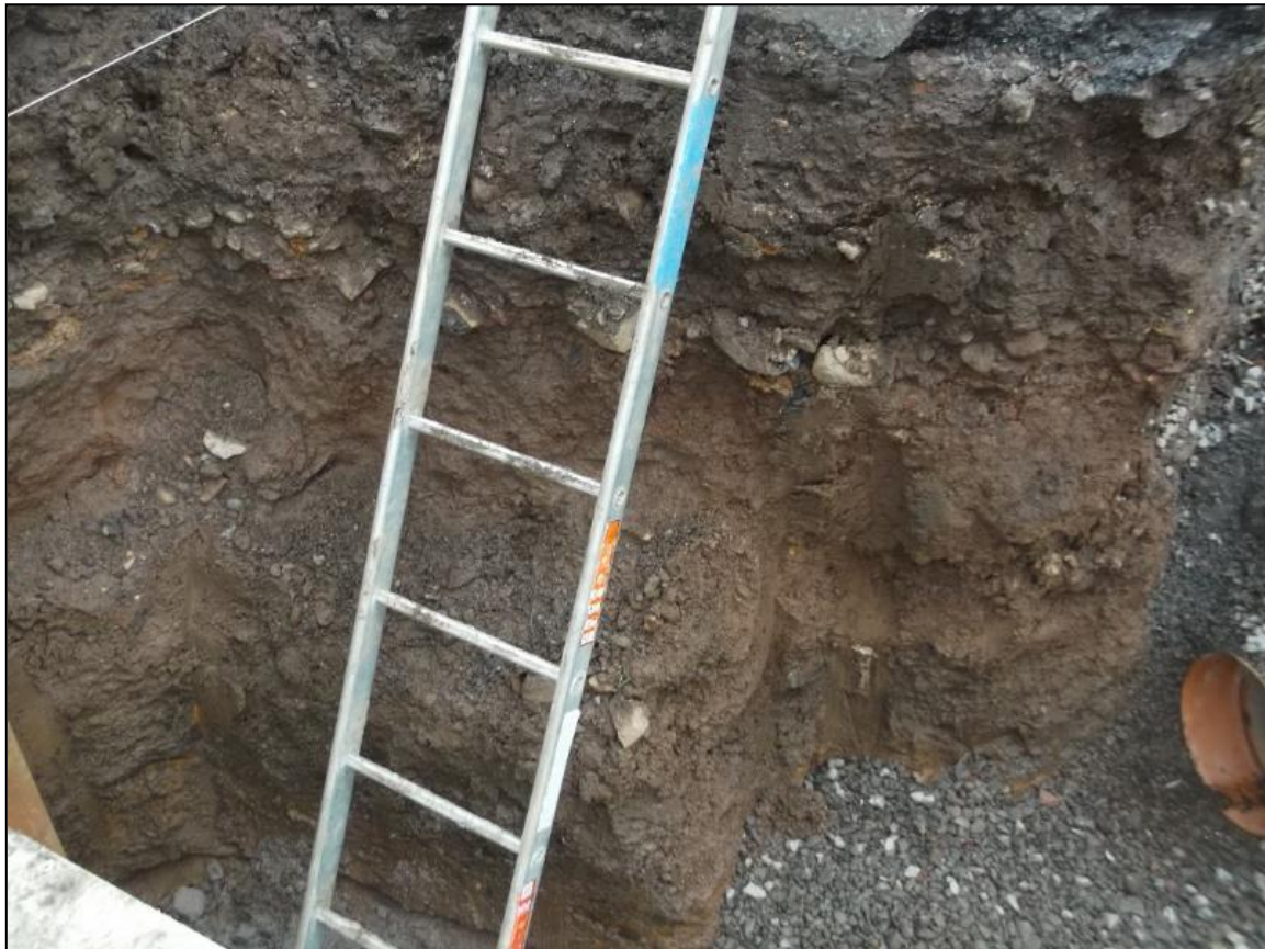
Figure 6b: Area 2 – Sample of southwest facing section
