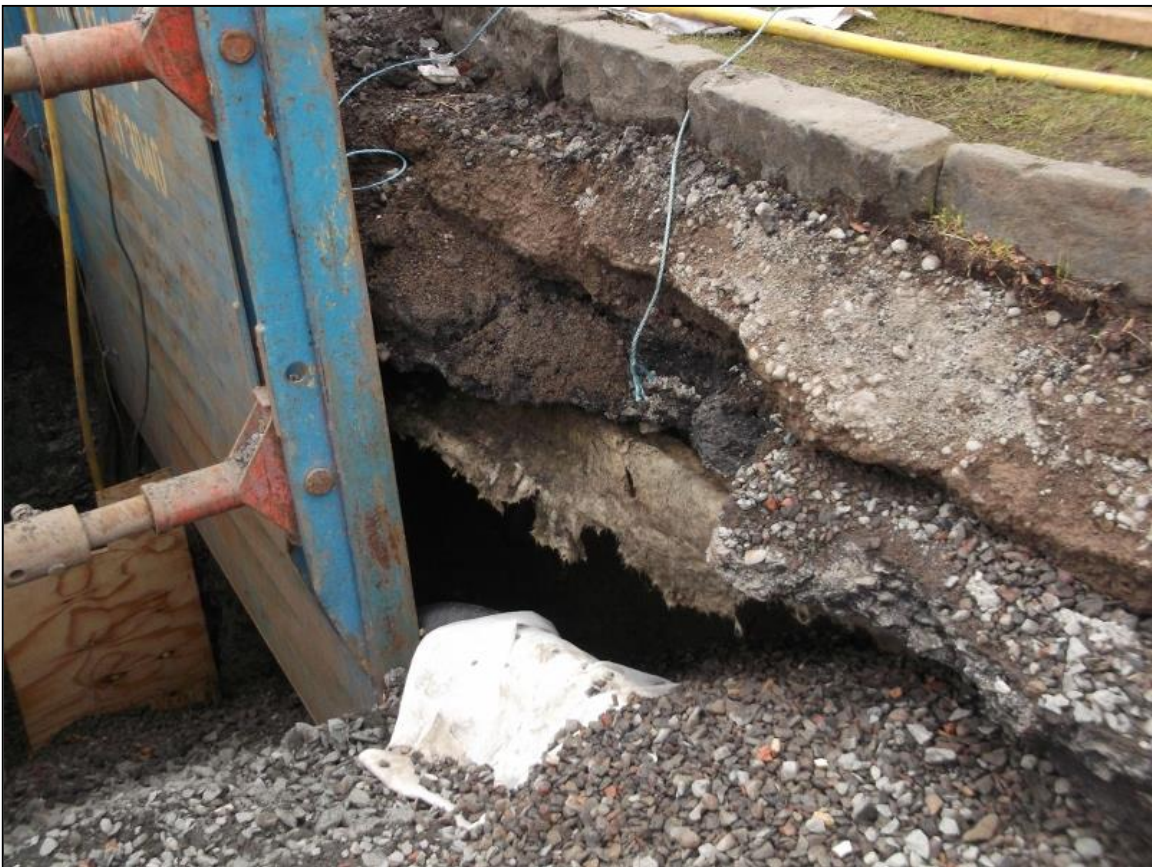
Figure 7b: Area 4 – shot showing depth of tarmac layers (007) and (008)
