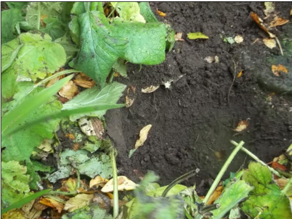
Figure 3b: Lightning Protection Works: Test Pit 2, Post excavation
