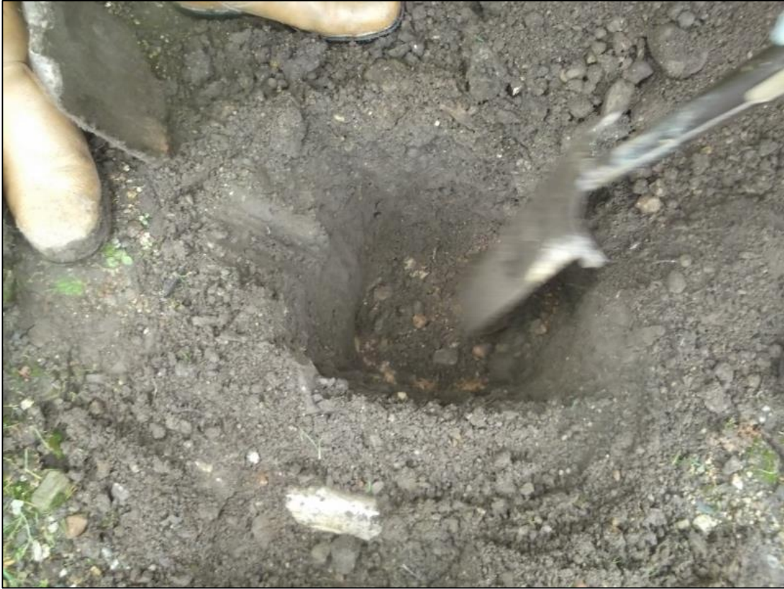
Figure 3a: Lightning Protection Works: Test Pit 1, Post excavation
