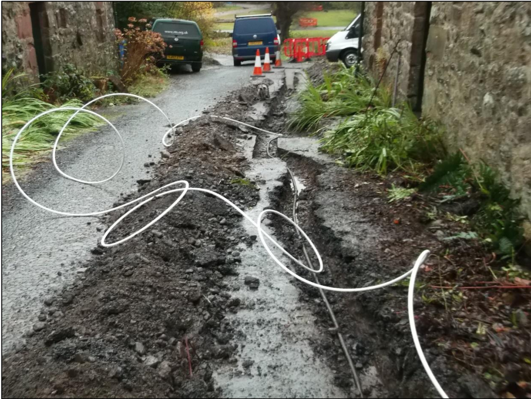
Figure 6a: General shot showing excavations along the road, from west-north-west
