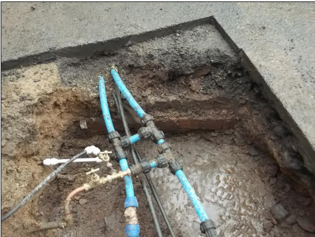
Figure 7b: Trench h, view of sandstone drain or culvert (010) from north
