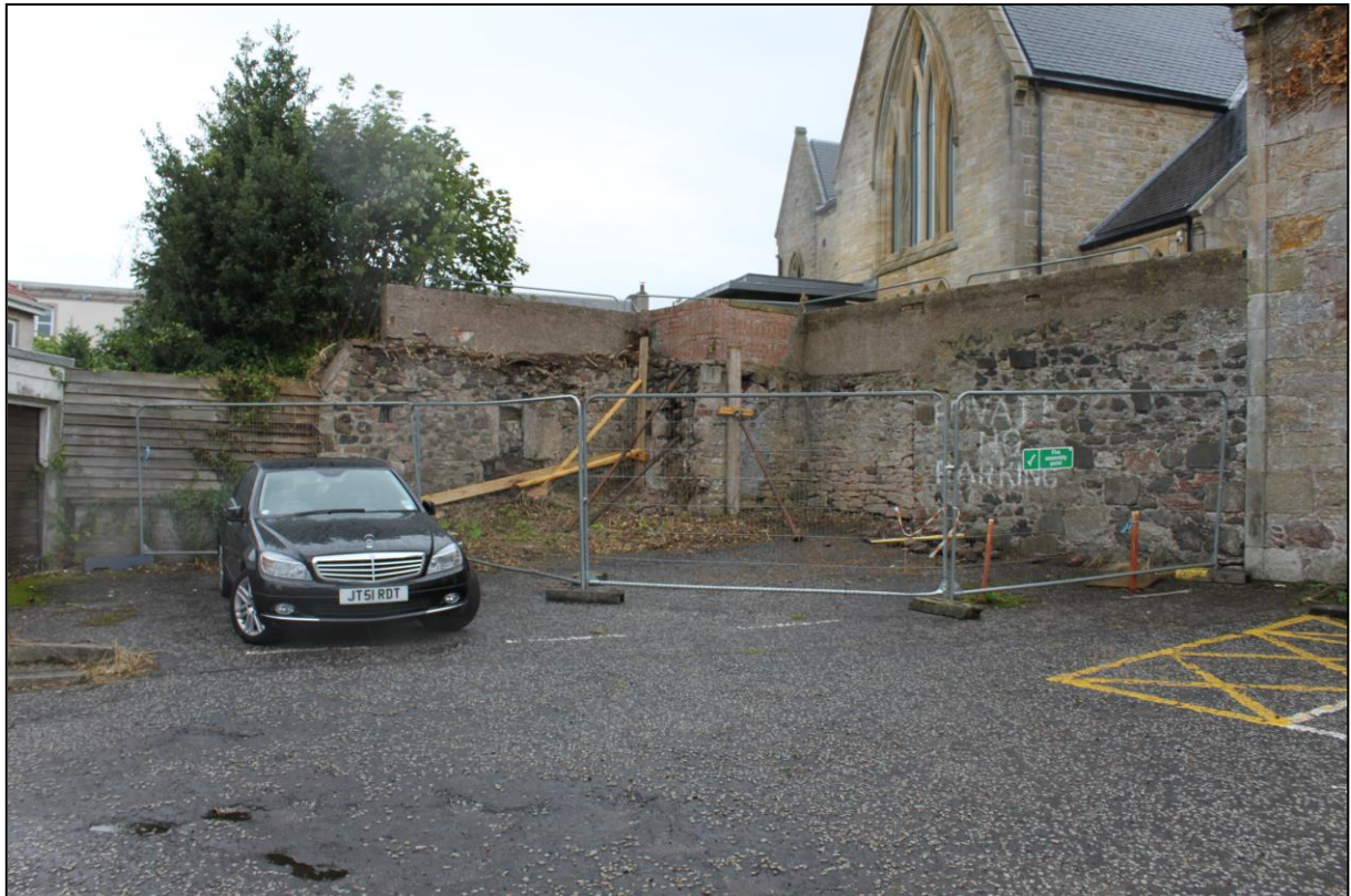
Figure 3: At time of Initial Site Inspection
