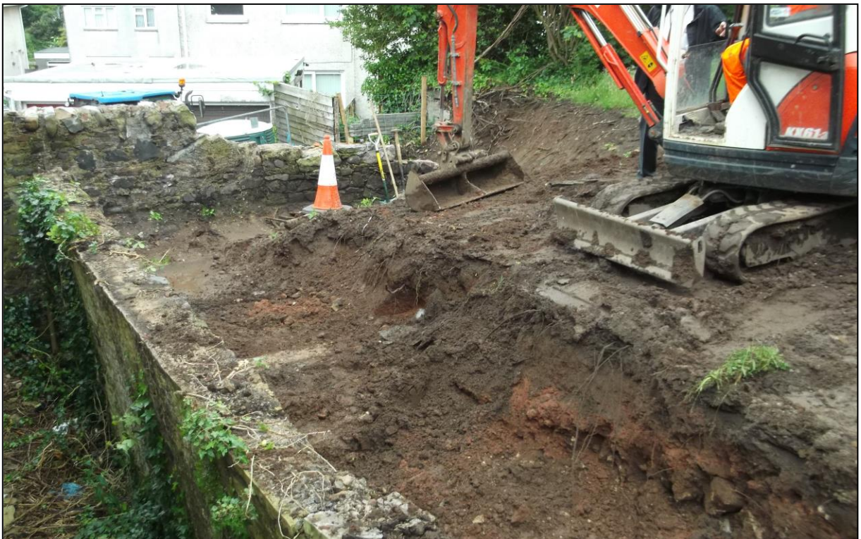
Figure 6: Monitored excavation revealing (501)
