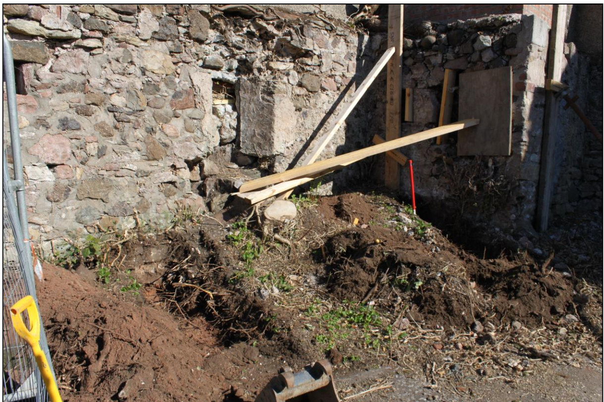
Figure 4: Detail of wall at time of Initial Site Inspection
