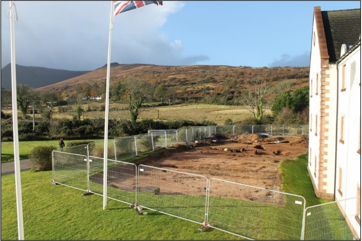
Figure 6a: General shot of site from the southeast
